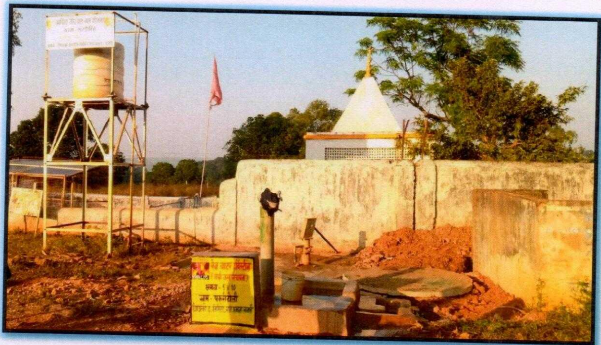
A View of Pond and RWH Structure
