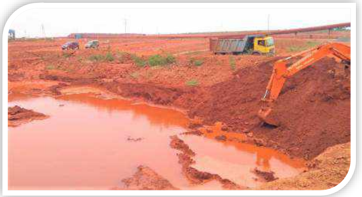
PHOTO 4: Showing Settling Pond Desilting
