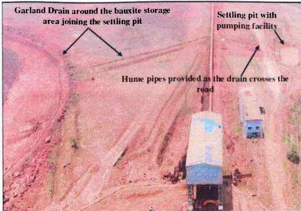
Figure 5: View of earthen retaining wall and garland drains near the bauxite storage area and crusher
