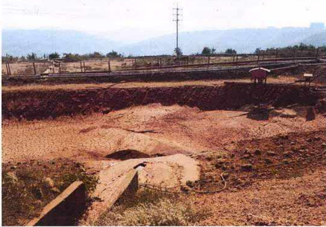
Figure 1: View of settling pit and pumps near the crusher
