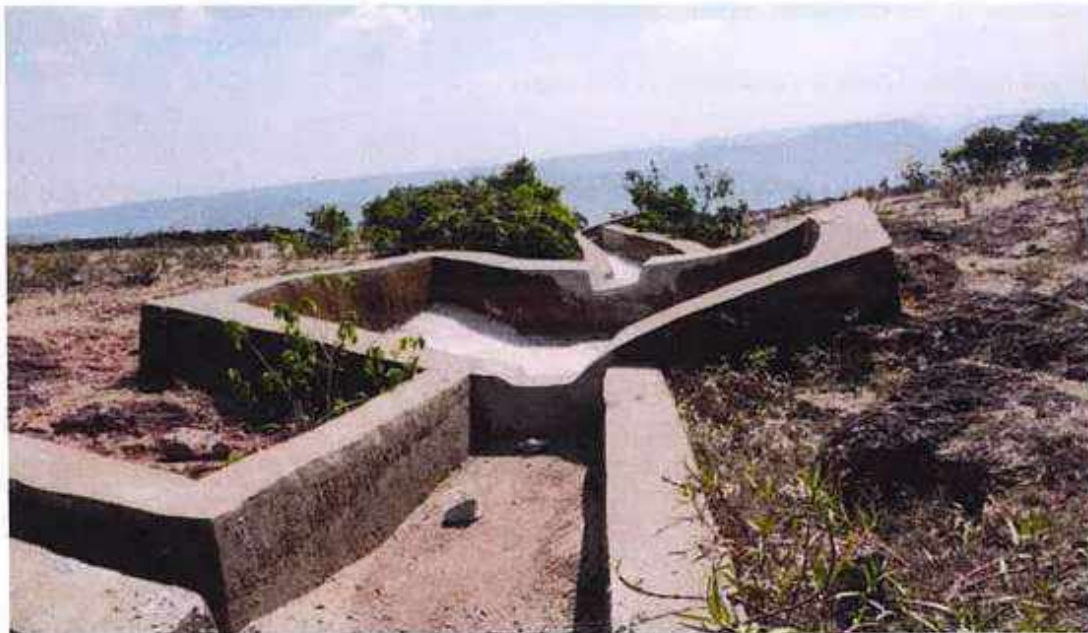
Figure 7: Renovated settling pits
