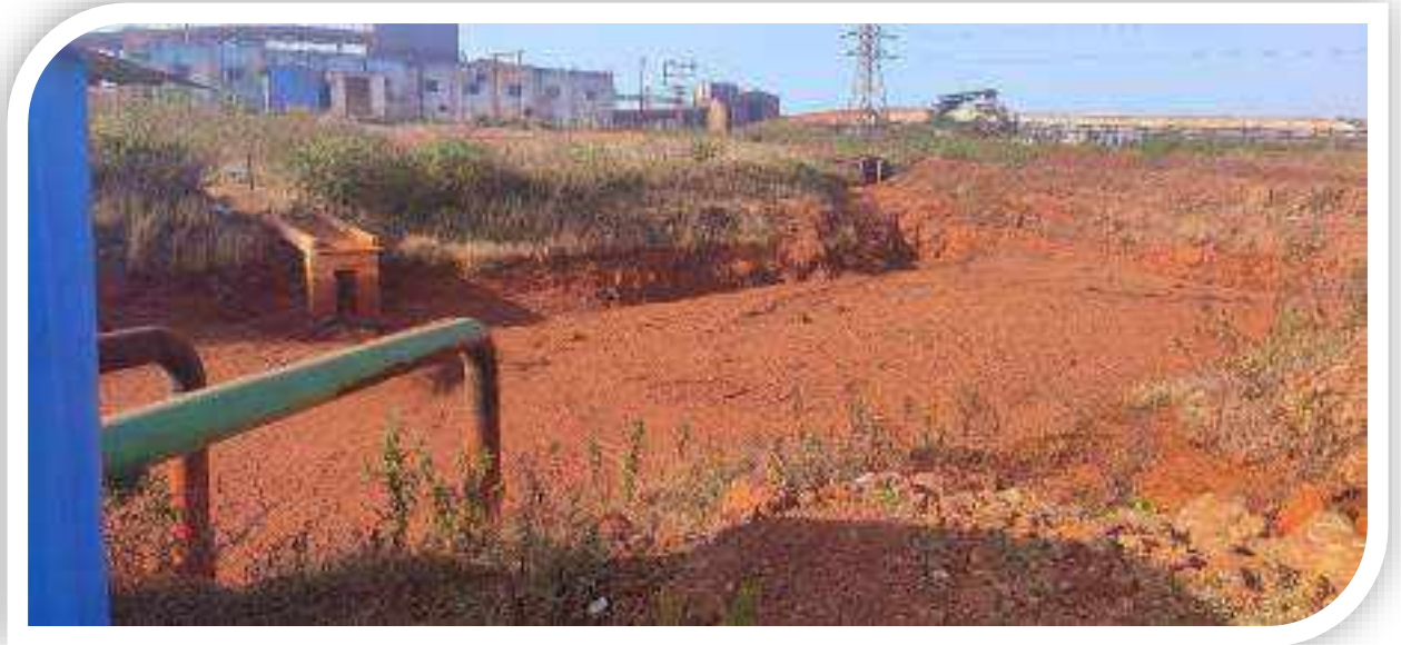
Settling Pond-2 Near Mines Entrance
