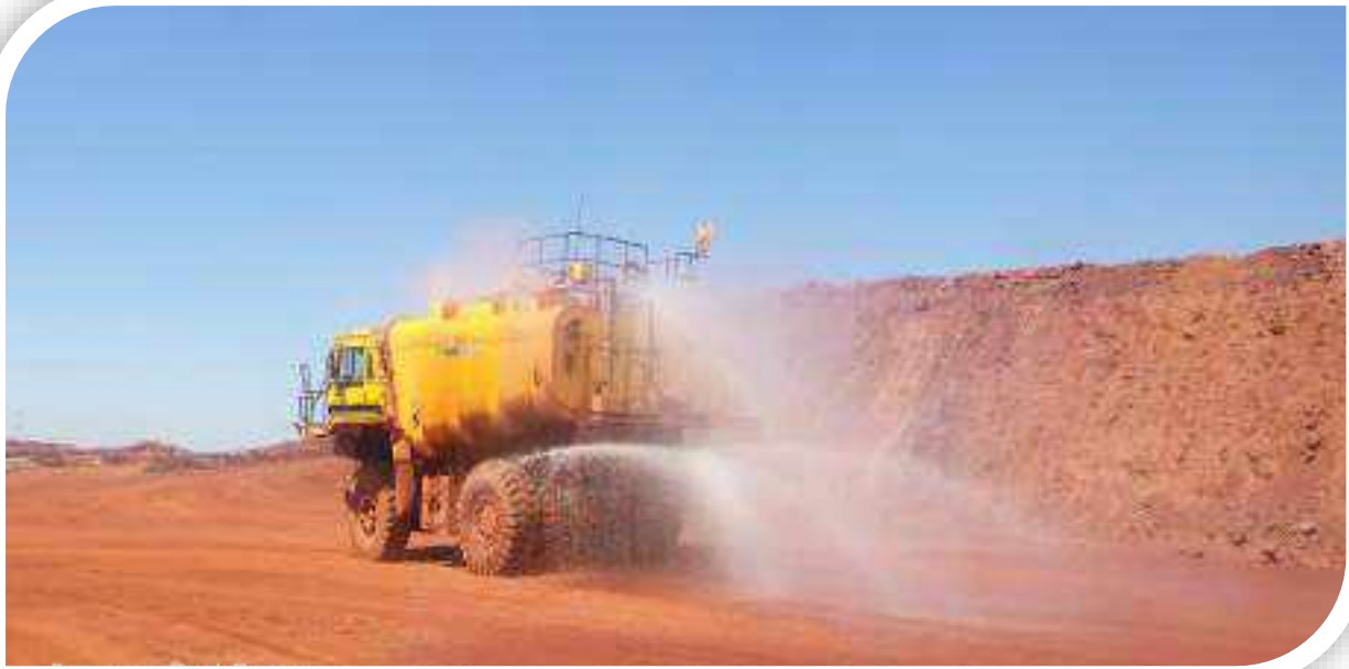
PHOTO 8: Showing 28KL Mobile sprinkler
