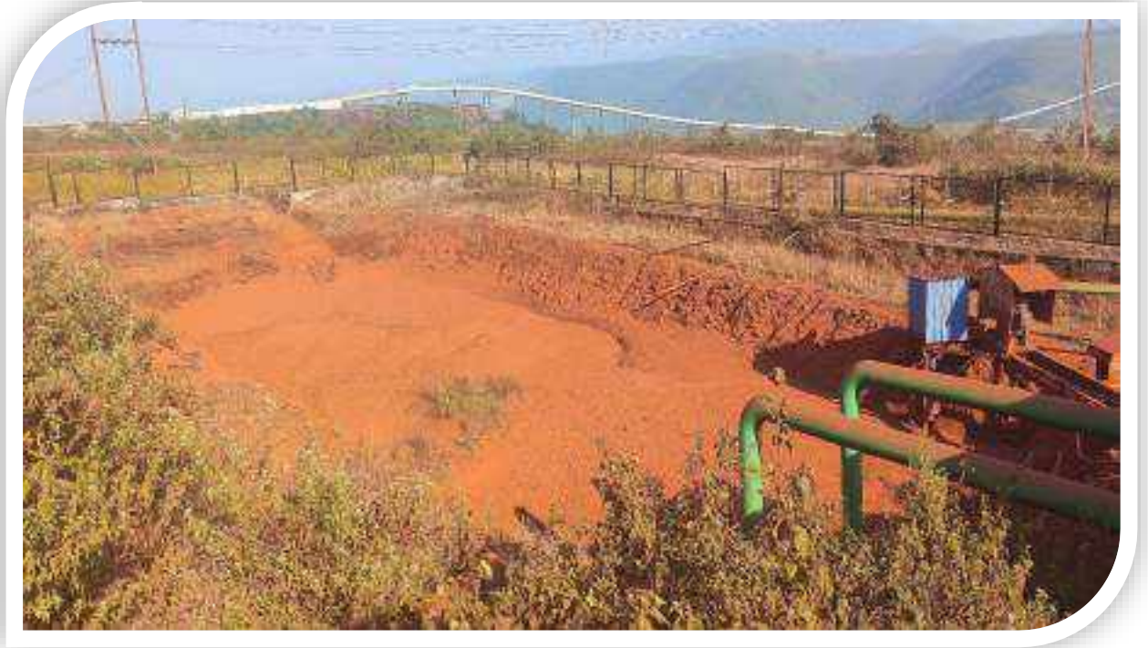
Settling Pit Near Crusher House
