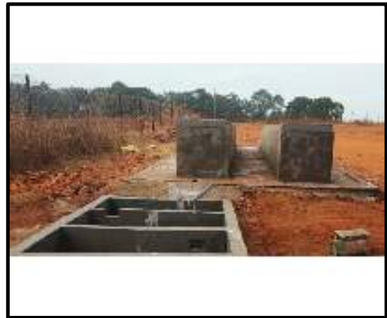
(Oil & Grease Trap – Washing Ramp)
