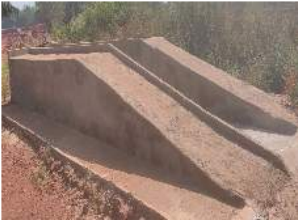
(Oil & Grease Trap – Washing Ramp)
