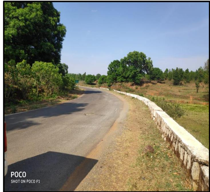
View of Black top road constructed up to pit head to reduce dust problem.
