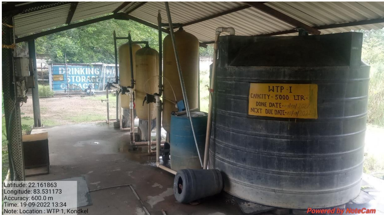
Water Treatment Plant (WTP) - 5 x 5 CuM per Hours
