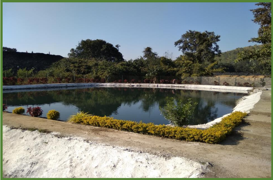
SETTLING POND NO – 2
