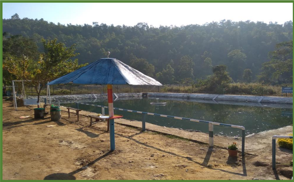
SETTLING POND NO – 3
