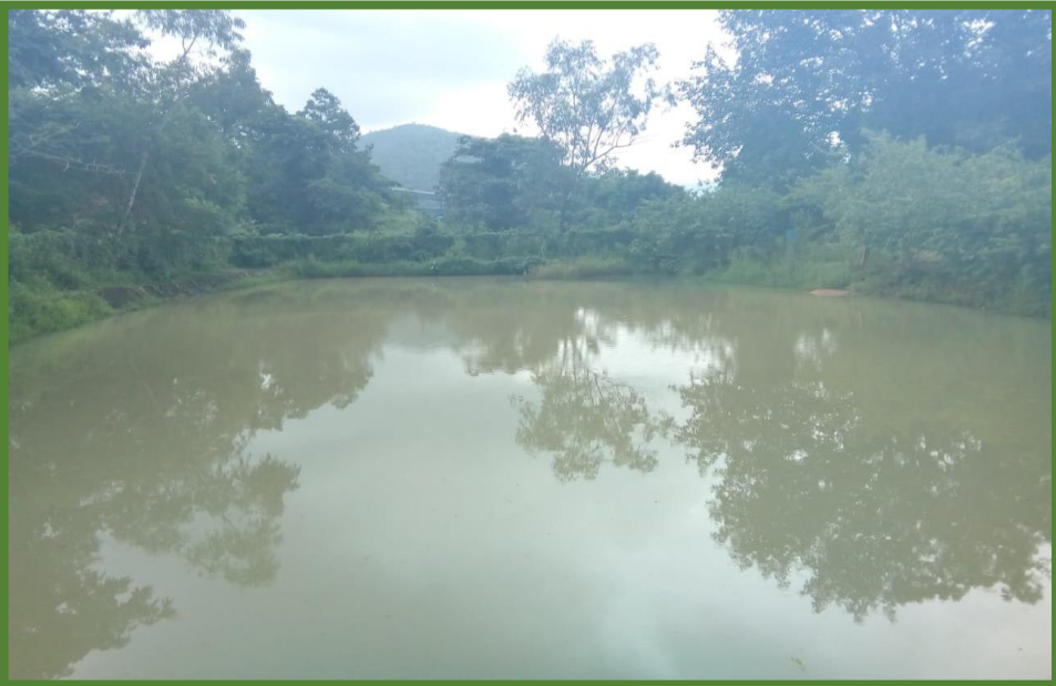
SETTLING POND NO – 1
