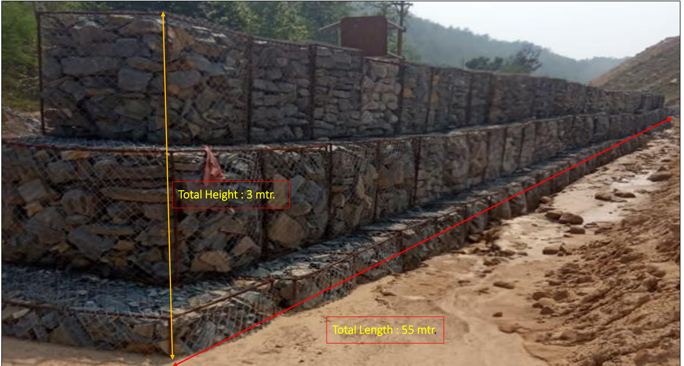
Gabion/Retaining wall at the toe of permanent dump slope for arresting the silt near Patch "C" in Banjikhoh, GP IV/4 Coal Mines.
