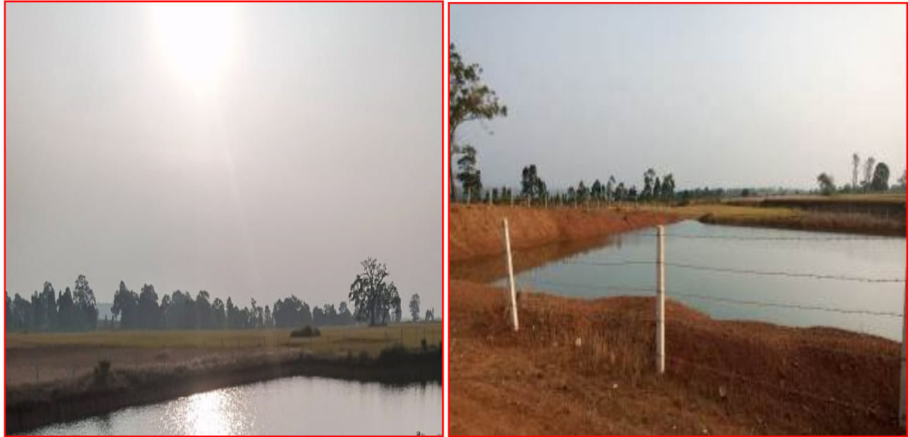
Rainwater Harvesting Pond at mines.
