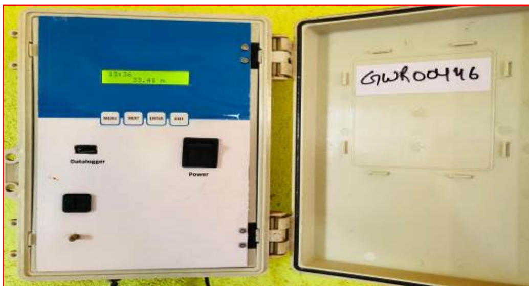
Piezometer Installed at Mines
