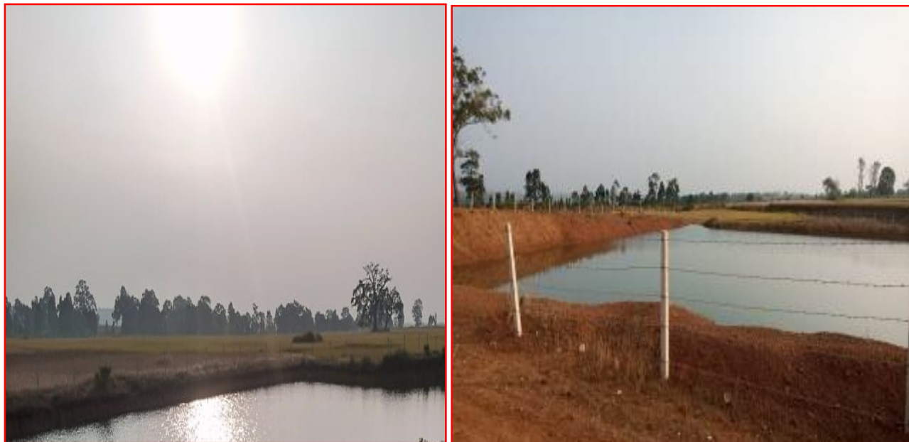
Rainwater Harvesting Pond at mines.
