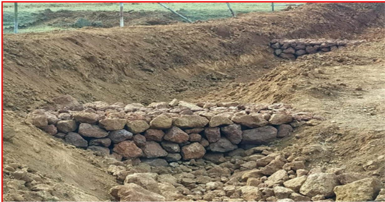
Catch drain Near mine pit.
