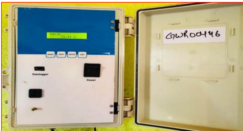
Piezometer Installed at Mines
