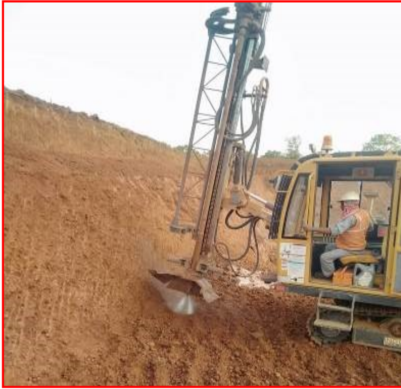
Wet drilling is being carried out.
