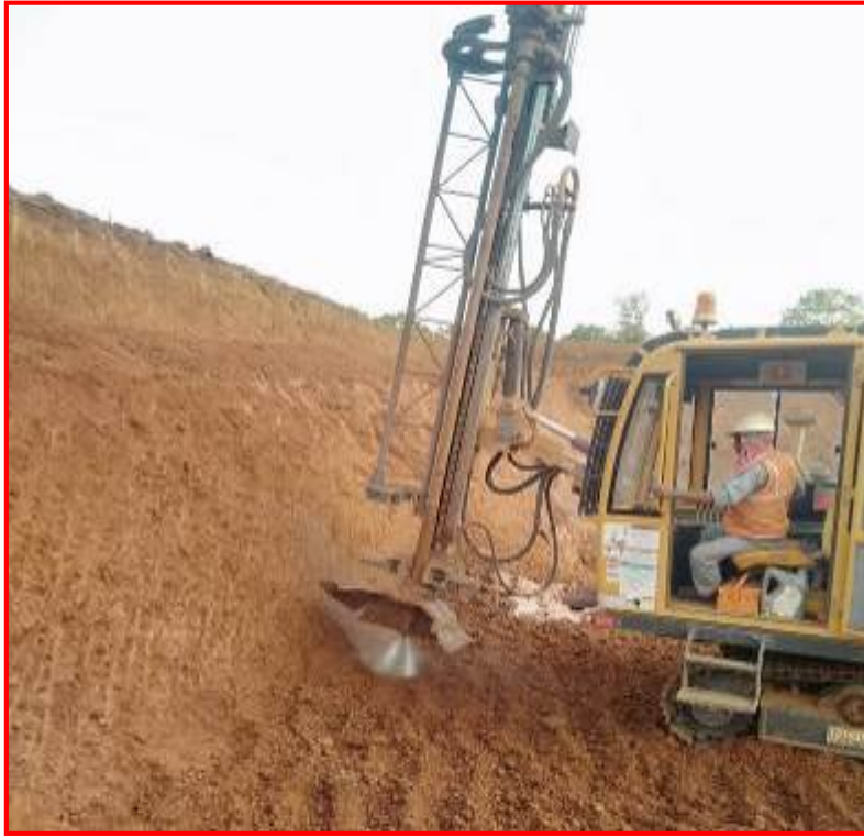
Wet drilling is being carried out.
