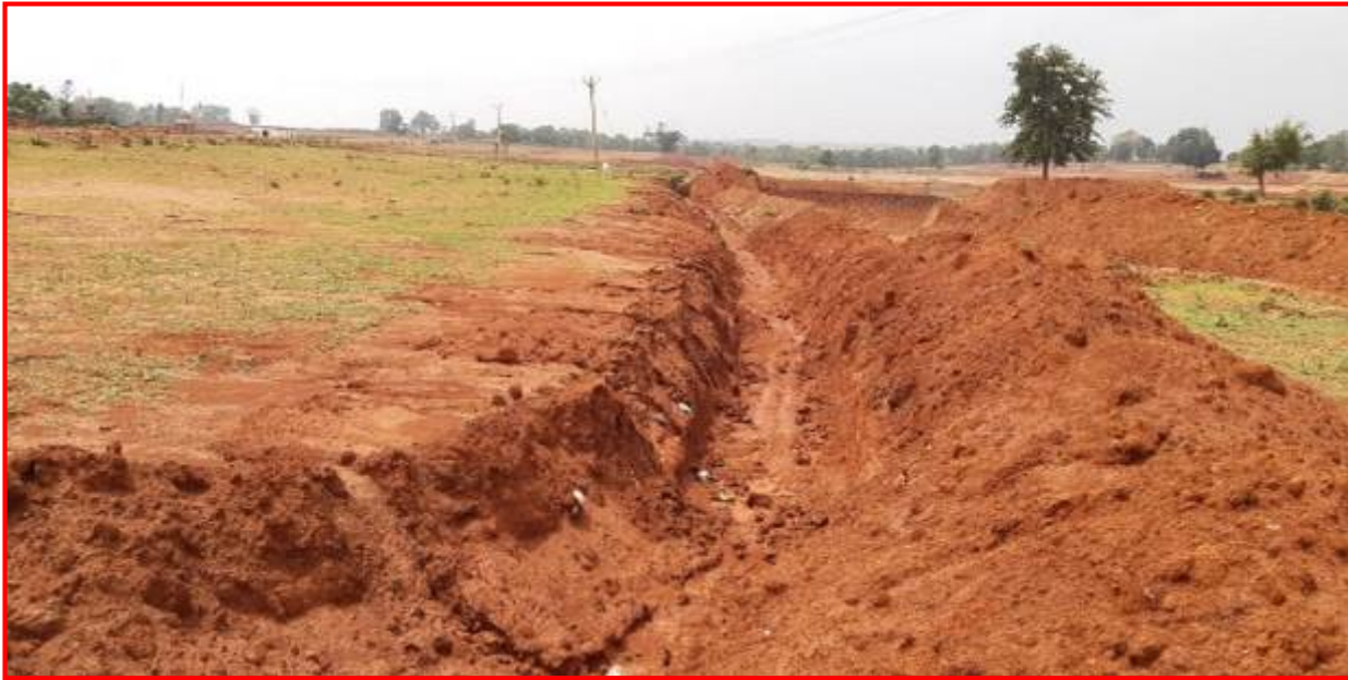
Garland drain around mine pit.
