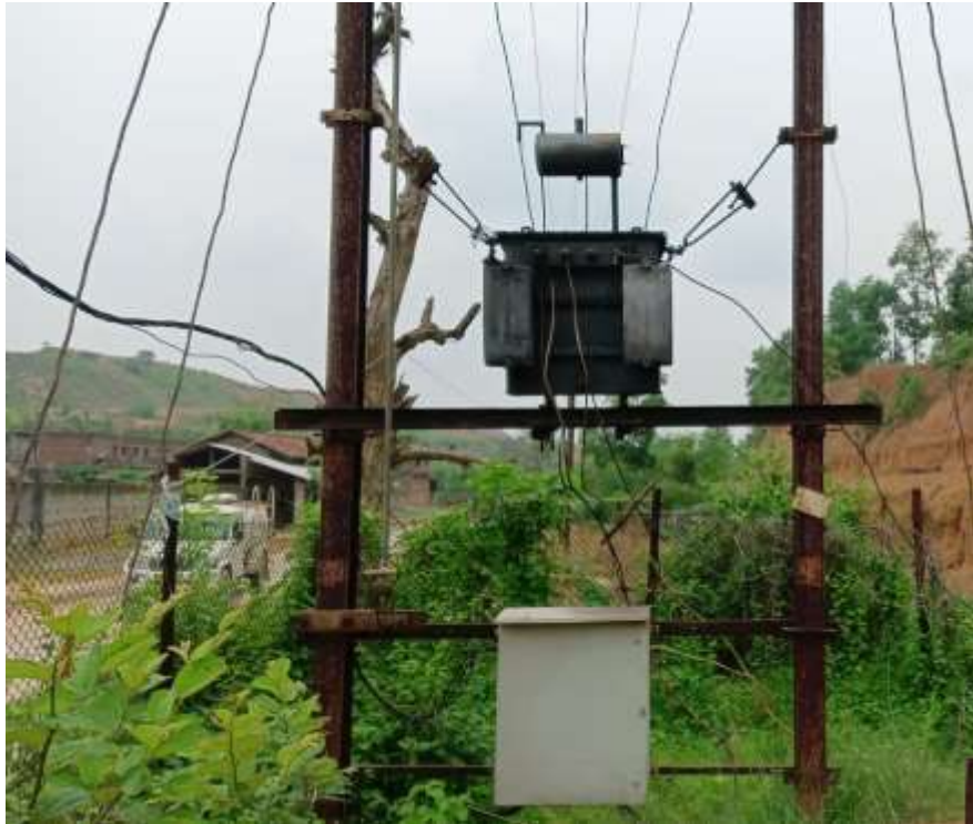
Installed Transformer
