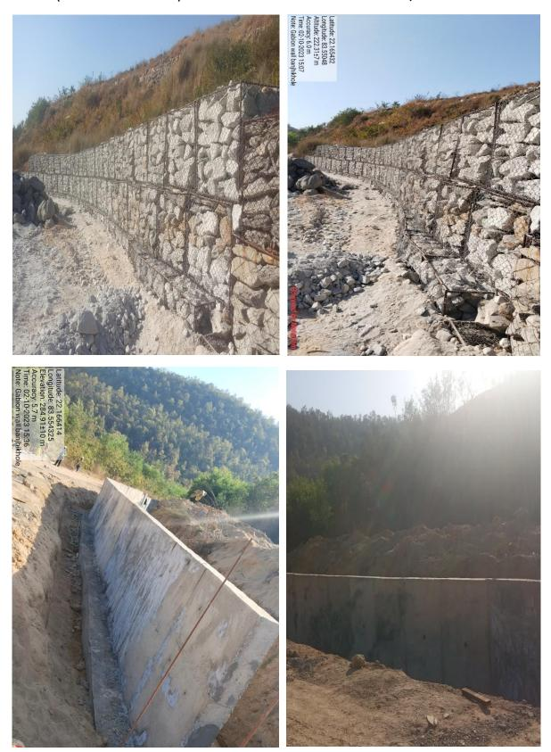
Total 50 m gabion/retaining wall constructed in 2<sup>nd</sup> Quarter (Aug'22 – Oct'22) at Patch "C" Banjikhol.
