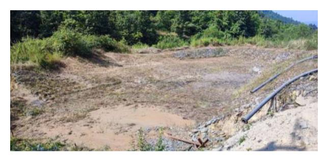
HIL constructed an additional settling pond of size 30m X 10m X 1.5m (01Nos) to collect whole mine seepage water generated during the mining activities from Patch "C" specially in the rainy season for proper settling of mine seepage water before discharge
