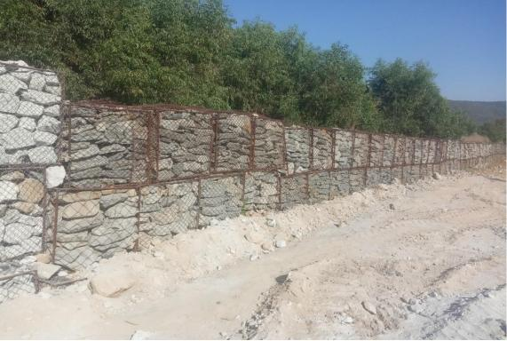
In the 1st Phase HIL has constructed approx. 55 mtr. long gabion/retaining wall at the toe of permanent dump slope near Patch "C" in Banjikhol, GP IV/4 Coal Mines.
