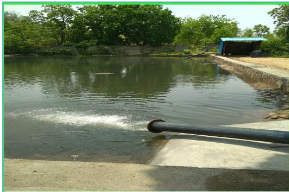
SETTLING POND NO – 5
