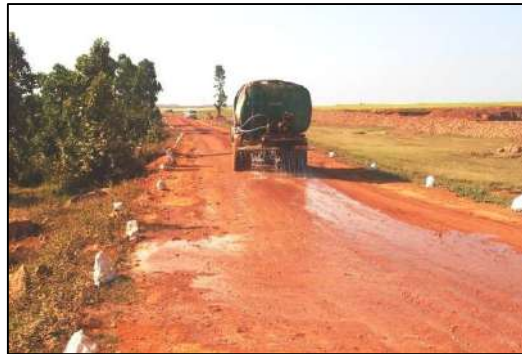
Water Sprinkling in the Haul Road
