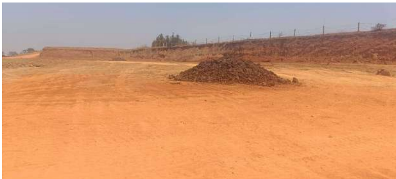
Land preparation for reclamation
