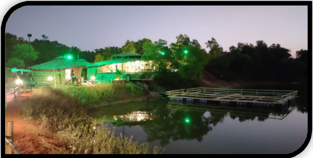
Rain Water Harvesting Pond
