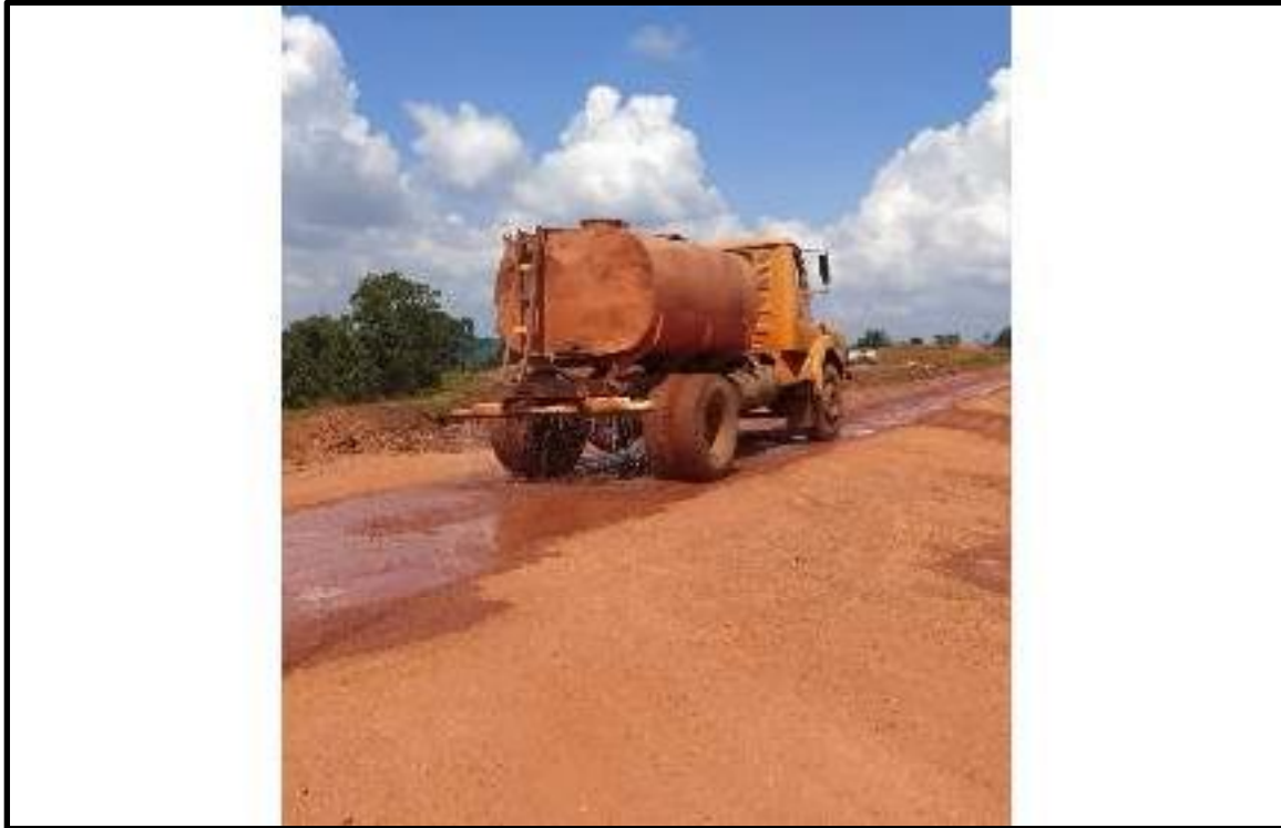
(Pic: Water sprinkling on mines haul road)
