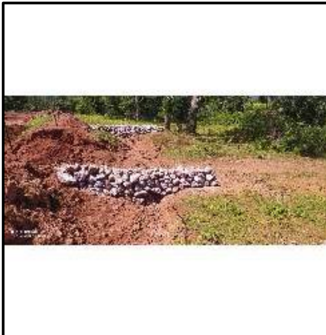
Pic: Garland drain, check dam & Retaining Wall
