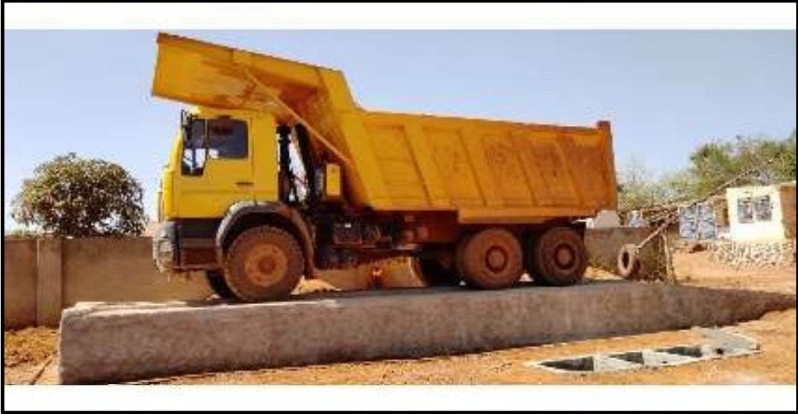
(Pic: Washing platform and oil & grease trap)
