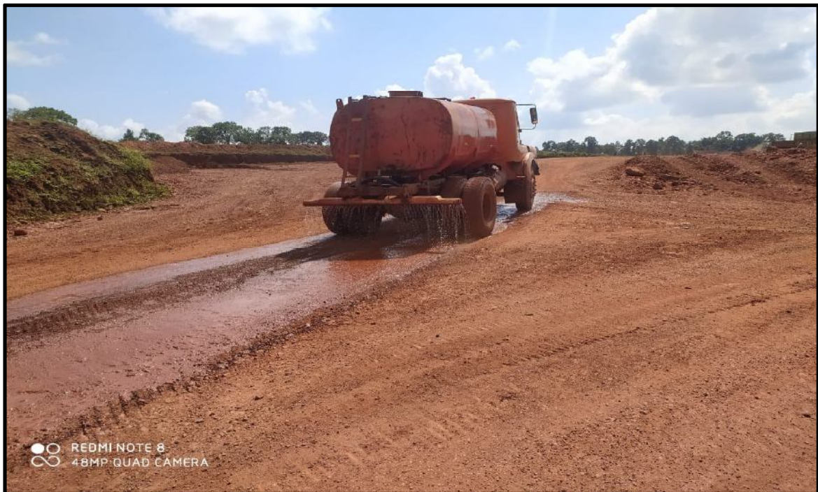
(Pic: Water sprinkling on mines haul road)
