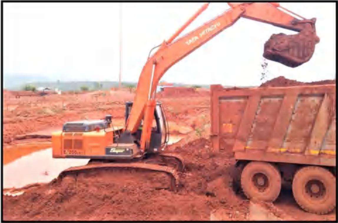
PHOTO 4: Showing Settling Pond Desilting
