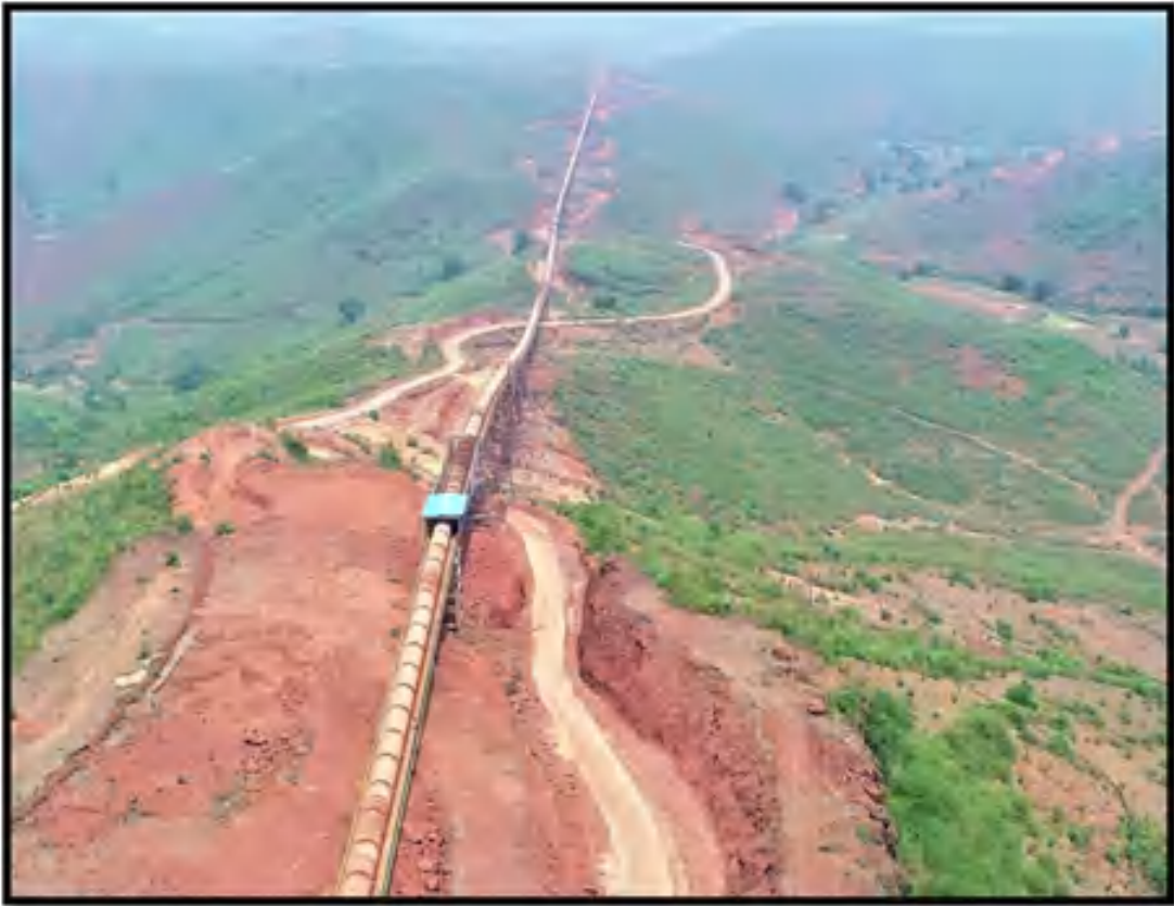
PHOTO 12: Showing Covered Long distance Conveyor
