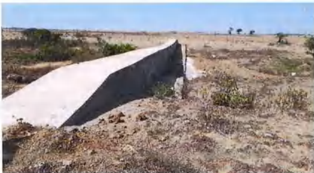
Figure 9b: Photographic view of the reconstructed check dam
