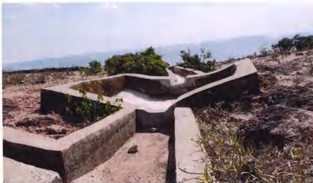
Figure 7: Renovated settling pits
