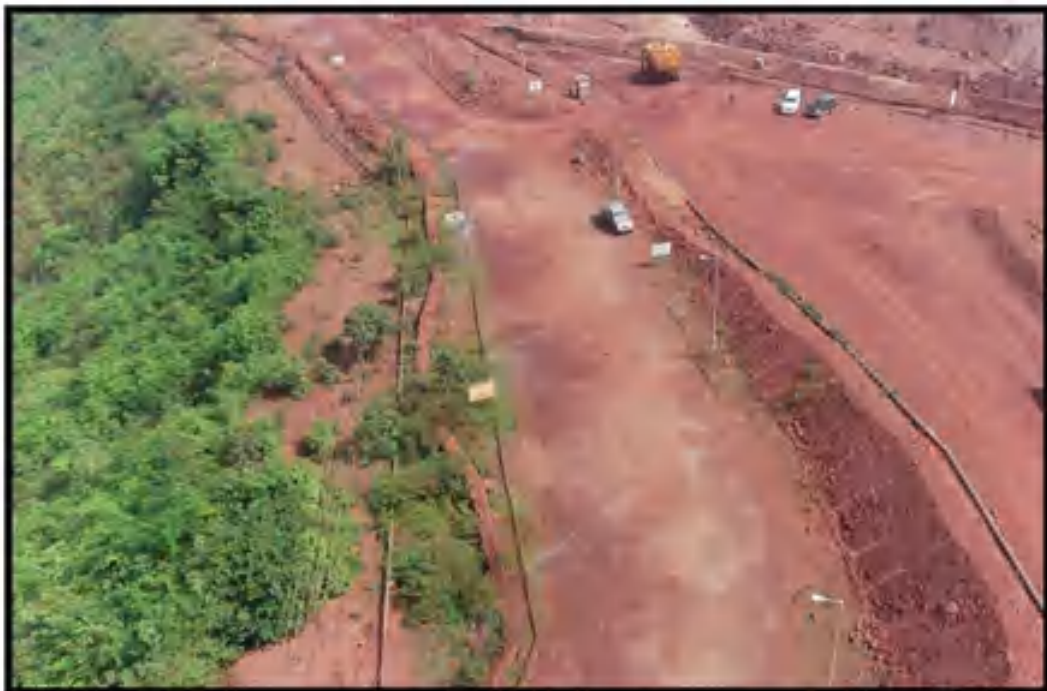
PHOTO 9: Showing Fixed Sprinklers
