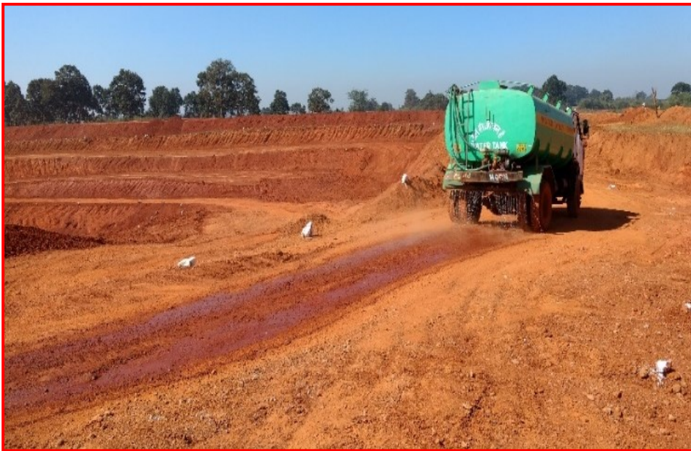
Mobile water tanker for dust suppression
