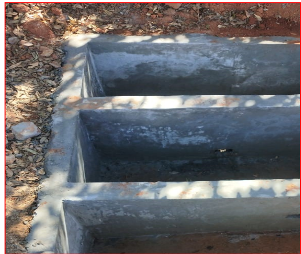
Oil and Grease Trap at Mines
