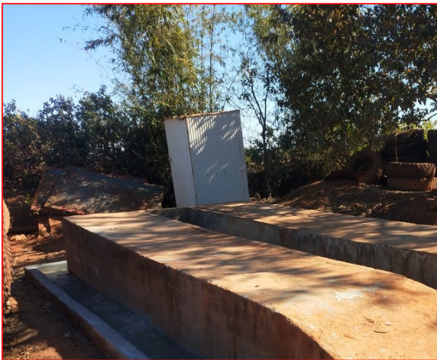
Oil and Grease Trap at Mines
