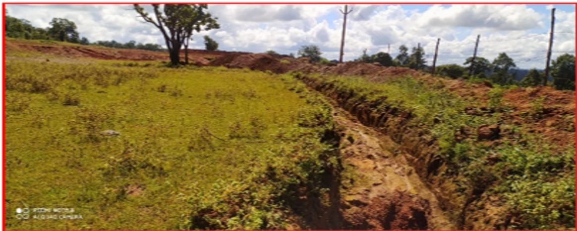
Garland drains around mine pit.
