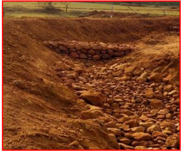
Retaining wall and siltation pit to prevent solid wash-
