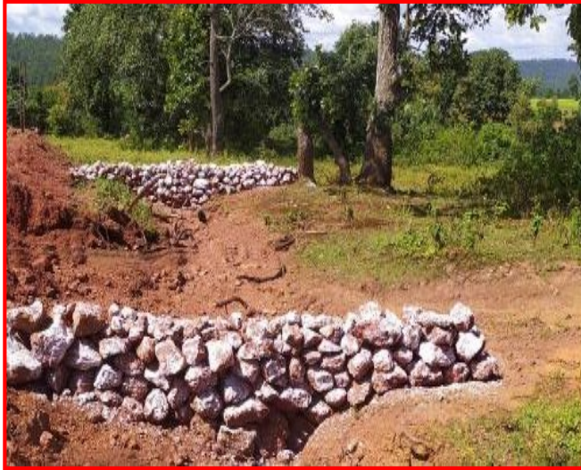
Retaining wall and siltation pit to prevent solid wash-
