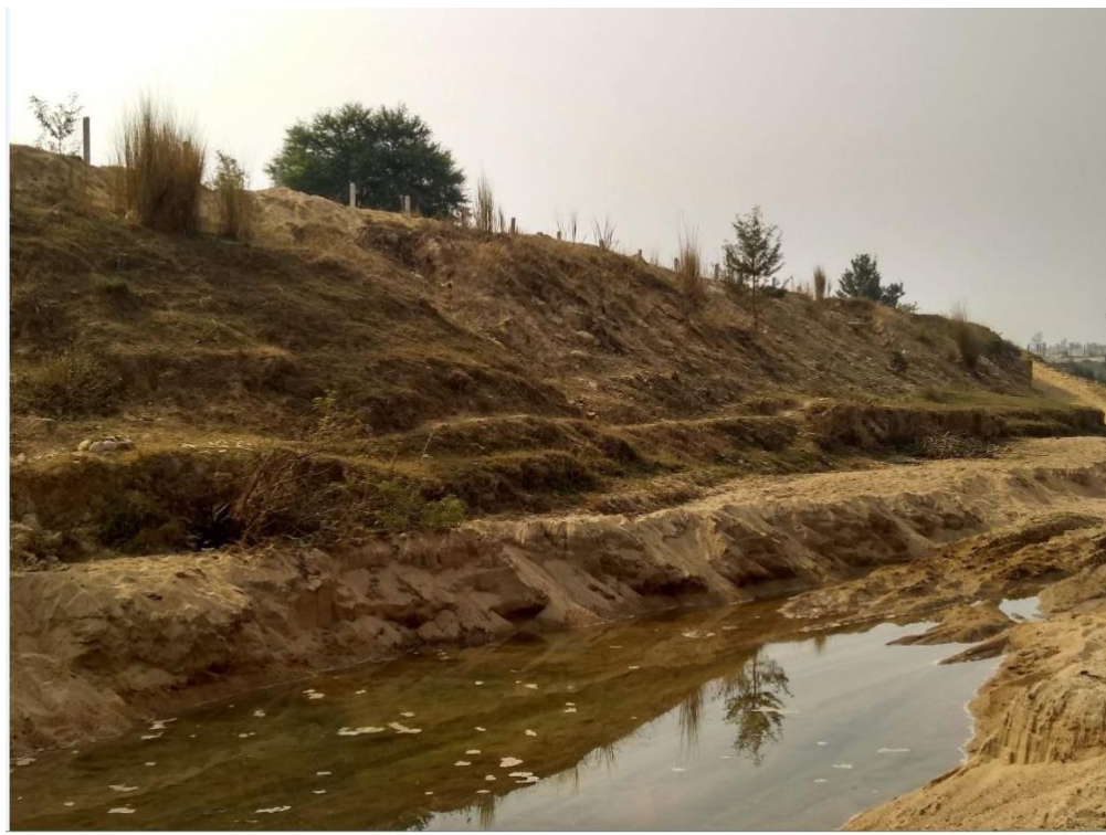
Figure 3: View of the embankment from the river bed
