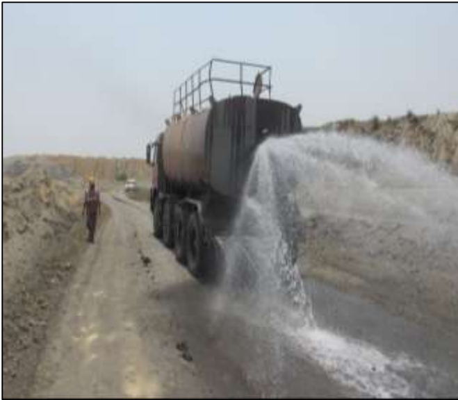
Figure 5: Water sprinkling by truck and Fixed Type Water Sprinkler for Dust Suppression
