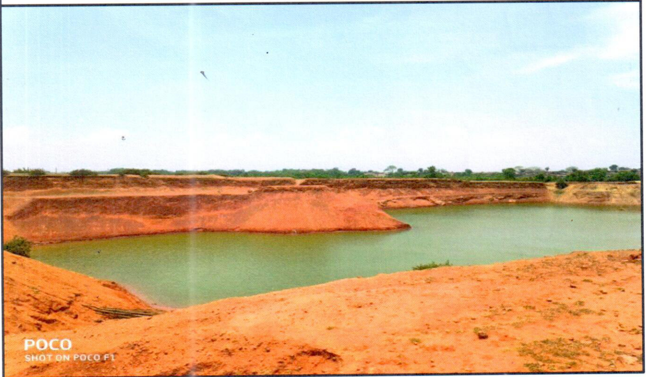
View of Recharge well and Pond
