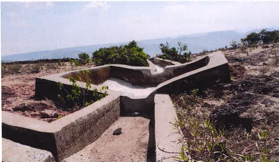
Figure 7: Renovated settling pits
