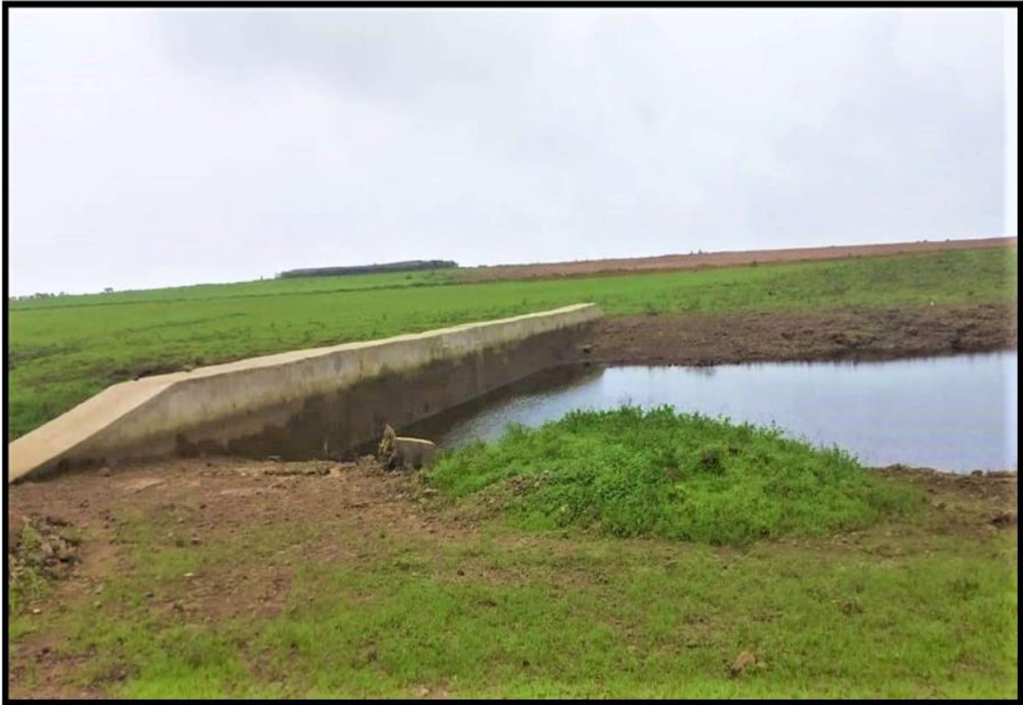
PHOTO 2: Showing Retaining wall & garland Drain along the Dump Slope
