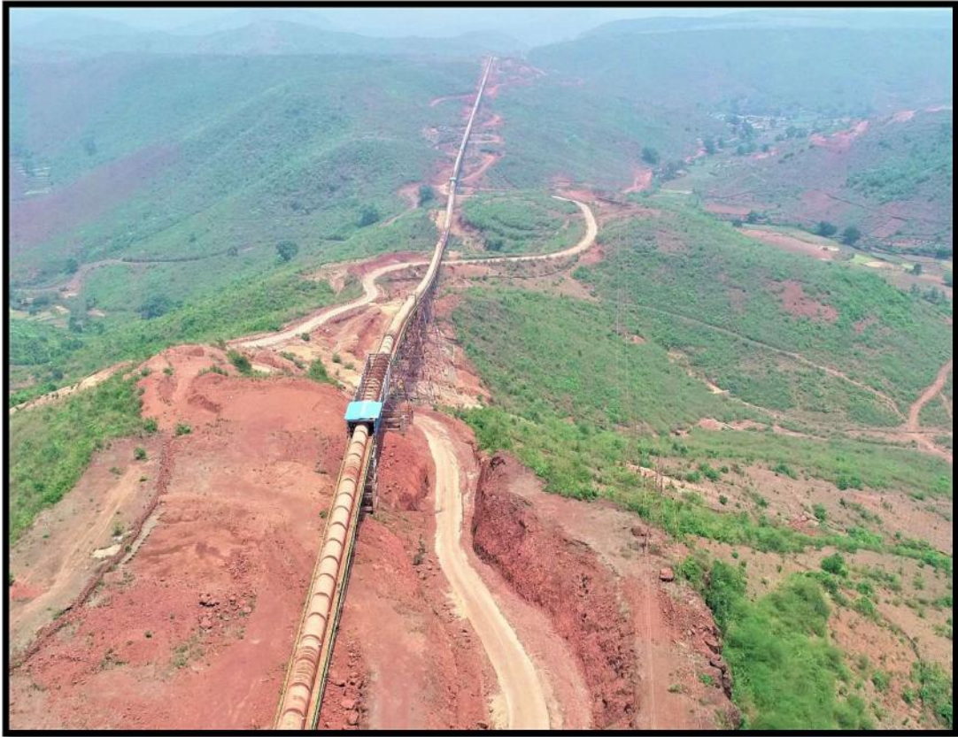
PHOTO 12: Showing Covered Long distance Conveyor
