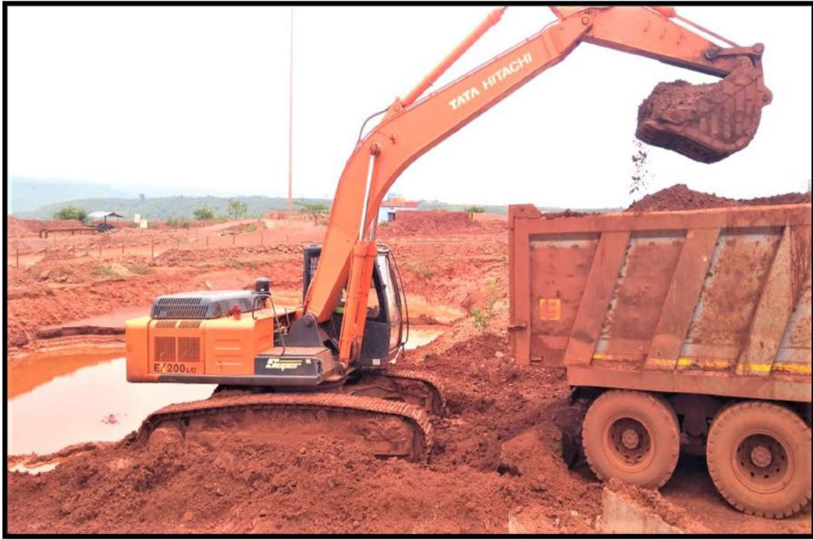
PHOTO 4: Showing Settling Pond Desilting
