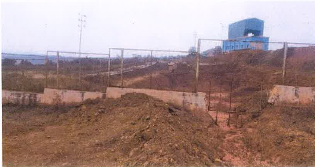
Figure 10: Fencing around the settling pit
