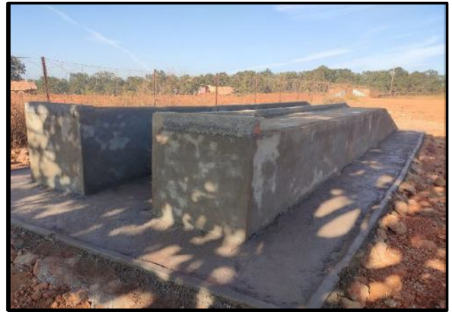
(Oil & Grease Trap – Washing Ramp)
