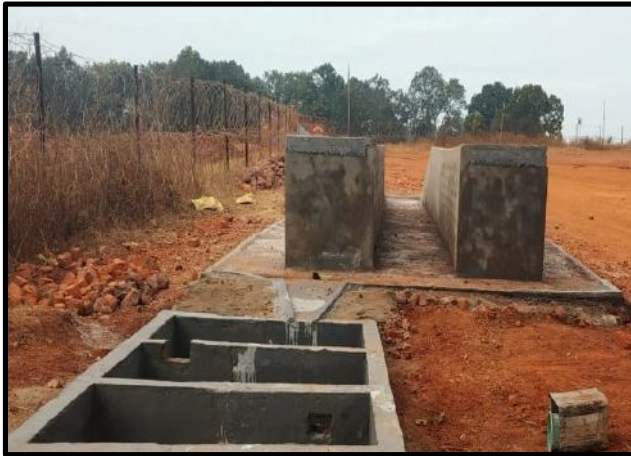
(Oil & Grease Trap – Washing Ramp)
