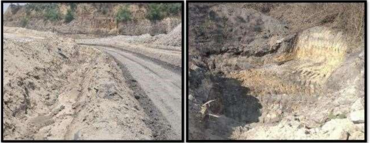
Fig 2- Garland Drain and Siltation Pond
