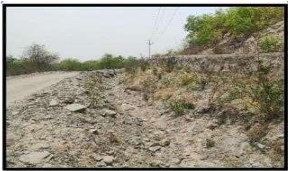
Fig 10 – Toe Wall along the Dump
