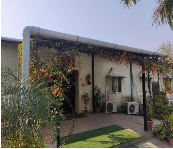
Fig 09 –Roof Top Direct Rainwater Harvesting Structure
