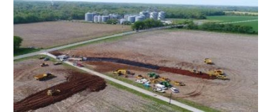
Broke ground May 2018 Guthrie, Kentucky
