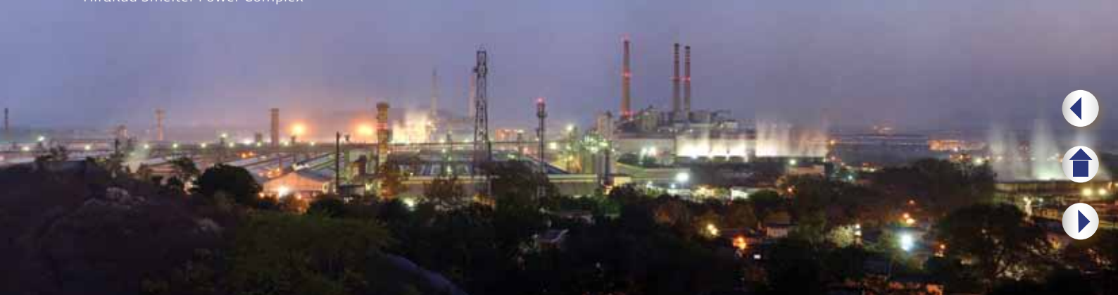
Hirakud Smelter Power Complex
