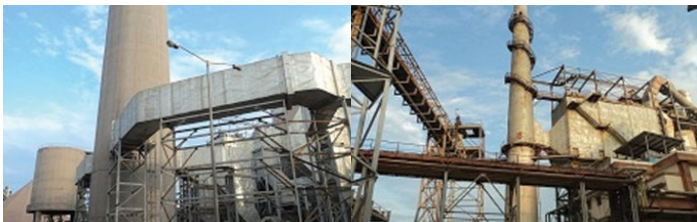
Air pollution control and management in Mahan Plant
