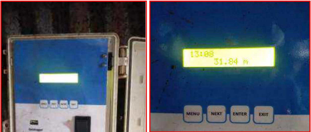
Installation of Piezometer at Kujam I Mine
