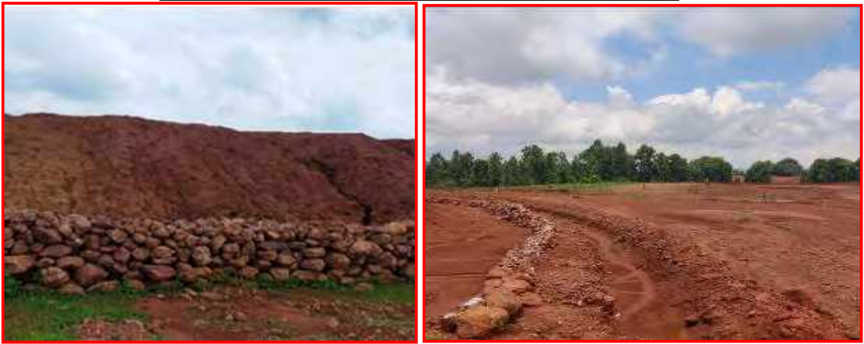
Retaining wall and Garland drain around mine pit.
