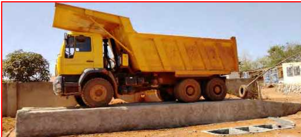
Washing ramp with Oil and Grease Trap
