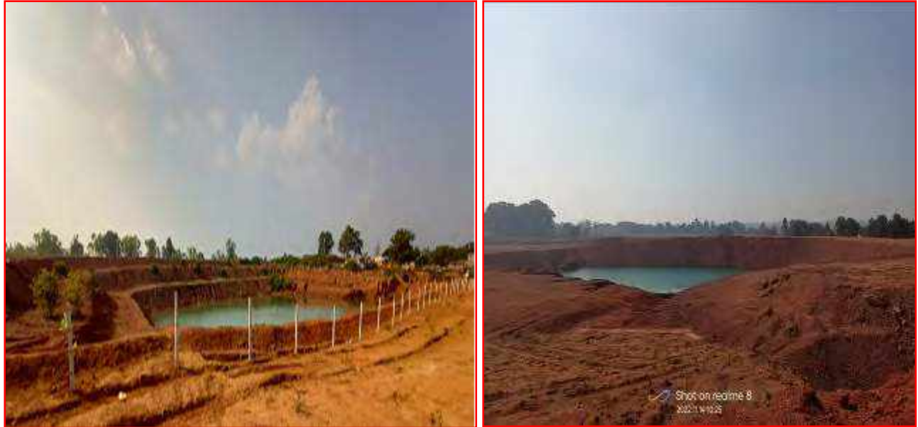
Rainwater Harvesting Pond in mines.
