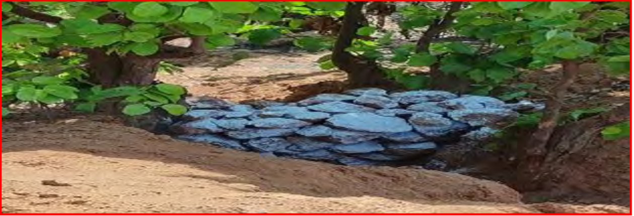
Retaining wall to prevent solid wash-off.
