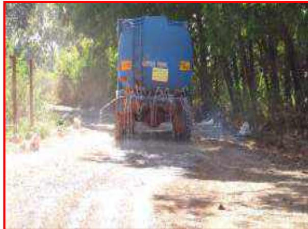
Water Sprinkling on Haul Road
