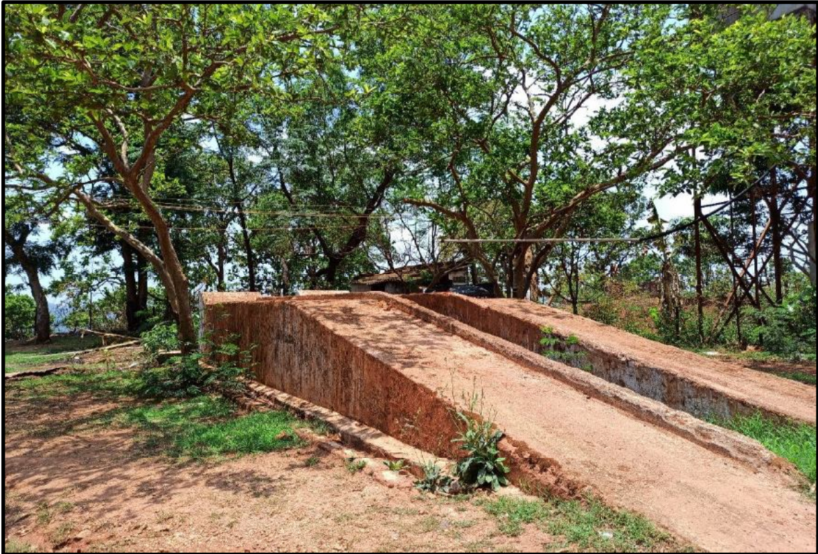
(Photographs of washing ramp and Oil and Grease Trap)
