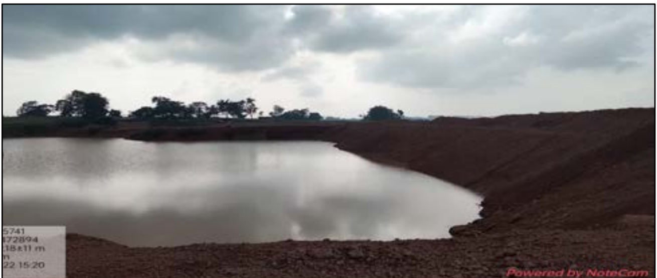
Rainwater Harvesting Pond
