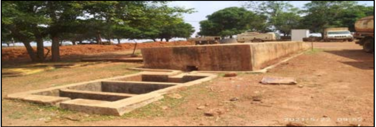
Washing Ramp and Oil and grease trap
