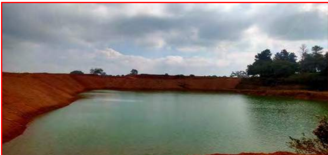
Rainwater Harvesting Pond
