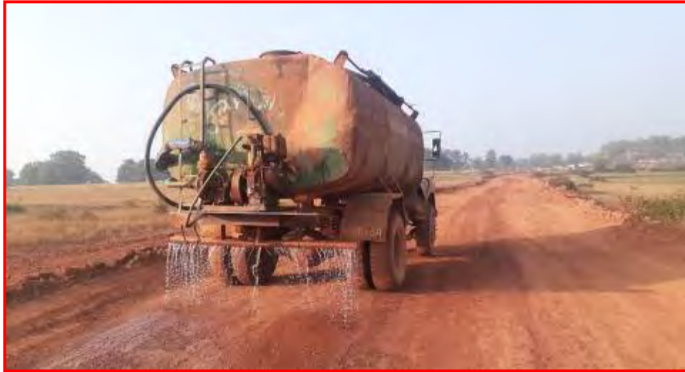
Dust Suppression through water tanker
