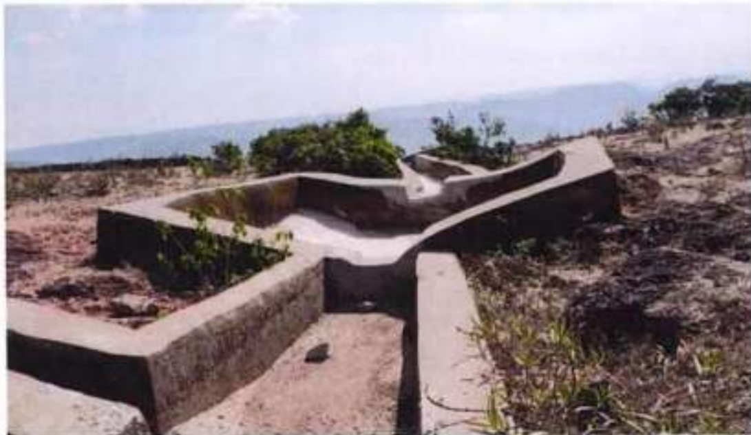
Figure 7: Renovated settling pits
