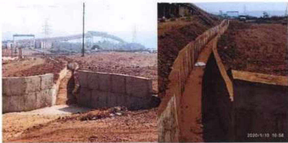
Figure 4: View of garland drains constructed in the R2 region
