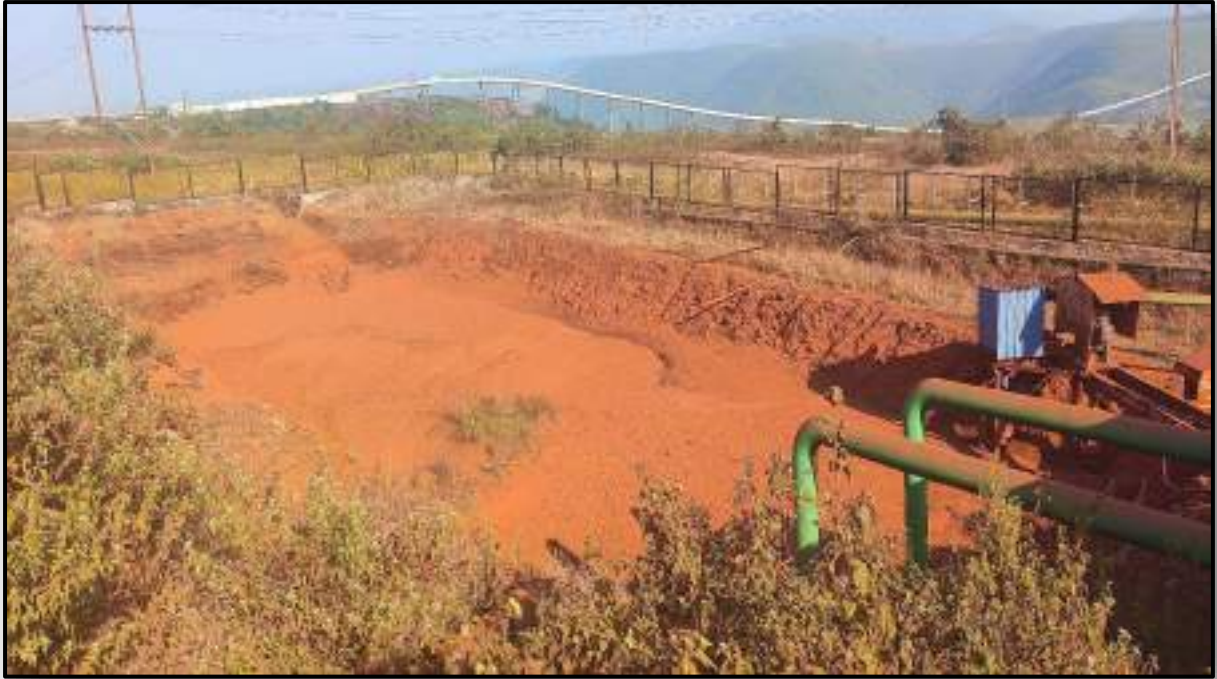
Settling Pit Near Crusher House
