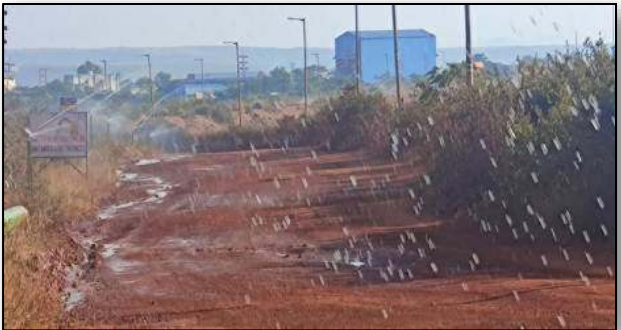
PHOTO 9: Showing Fixed Sprinklers
