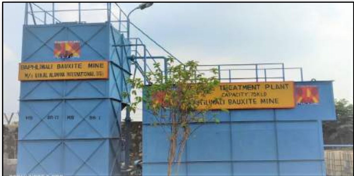
PHOTO 15: Showing 75 KLD Sewage Treatment Plant(STP)
