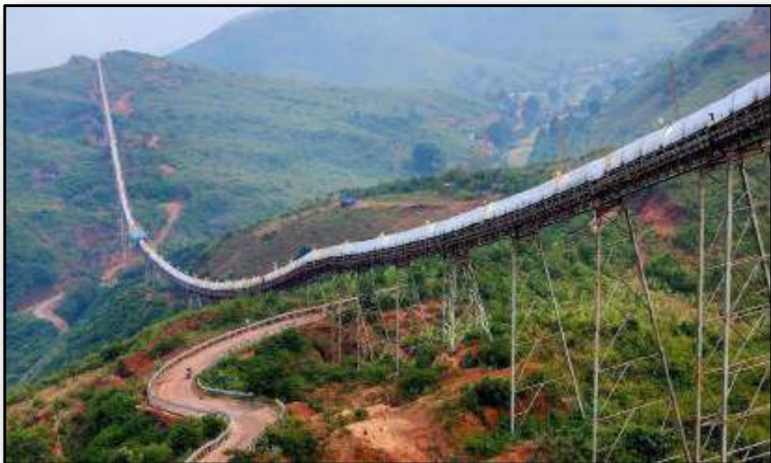
PHOTO 13: Showing Covered Long-Distance Conveyor (LDC)
