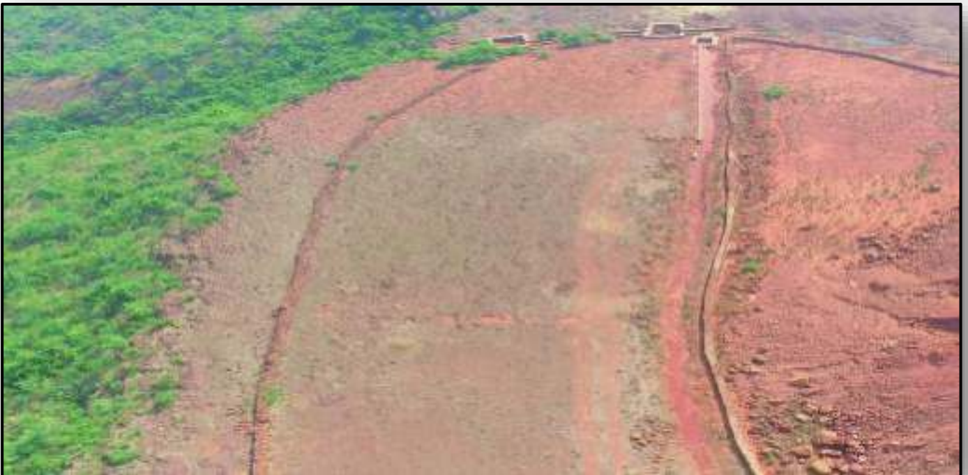
PHOTO 2: Showing Retaining wall & garland Drain along the Dump Slope
