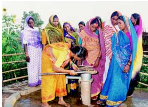
Hands pumps installed, operated & maintained by women in villages surrounding Renukoot.
