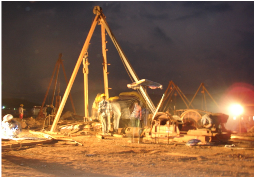
Non-plant buildings - Piling work in progress
