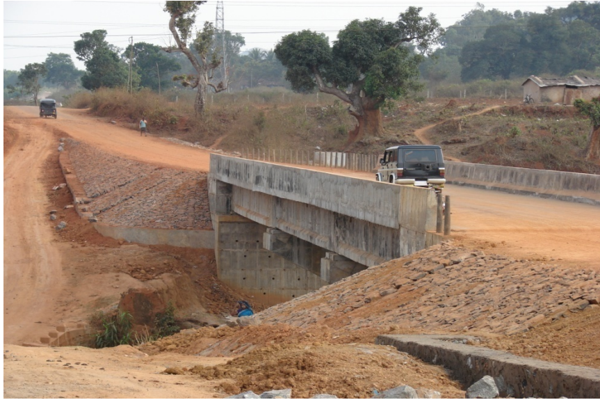
Laxmipur Bridge - open for vehicle traffic
