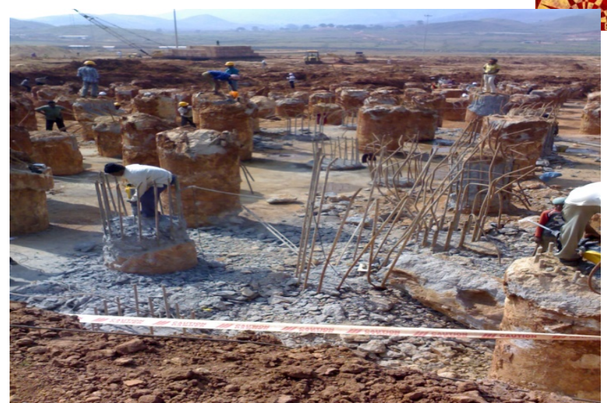
Precipitation Tanks - pile cap foundations under progress
