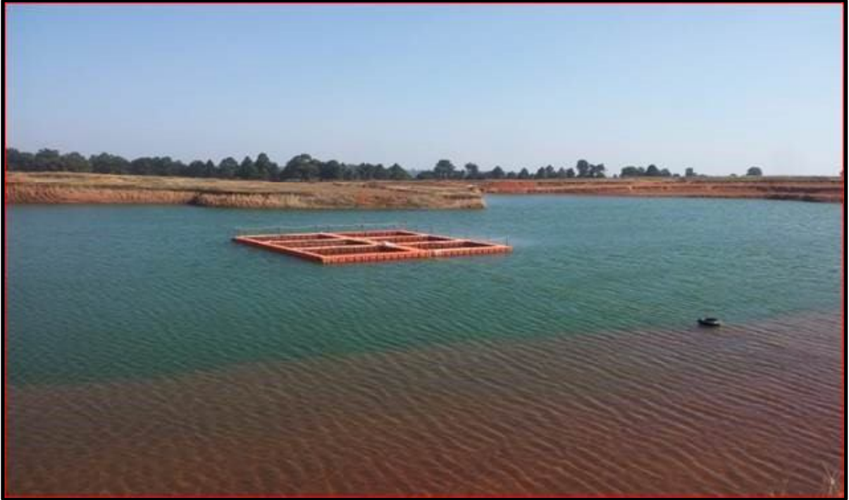
(Rainwater harvesting pond)
