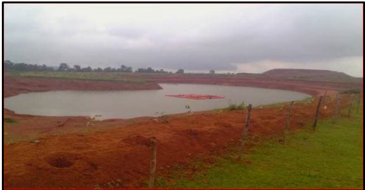
(Rainwater harvesting pond)
