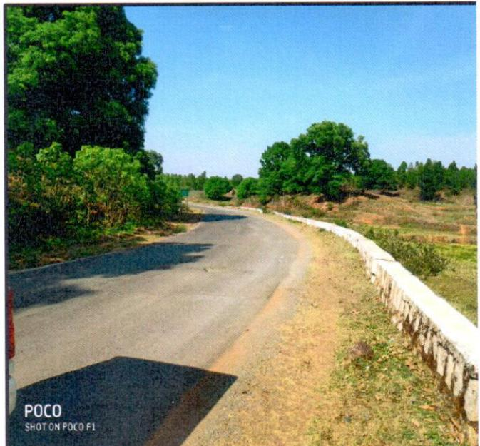
View of Black top road constructed up to pit head to reduce dust problem.
