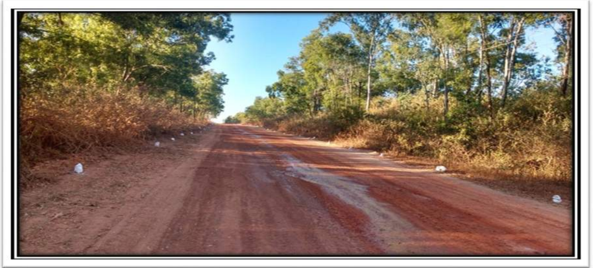
(Green Belt Development along Road side)
