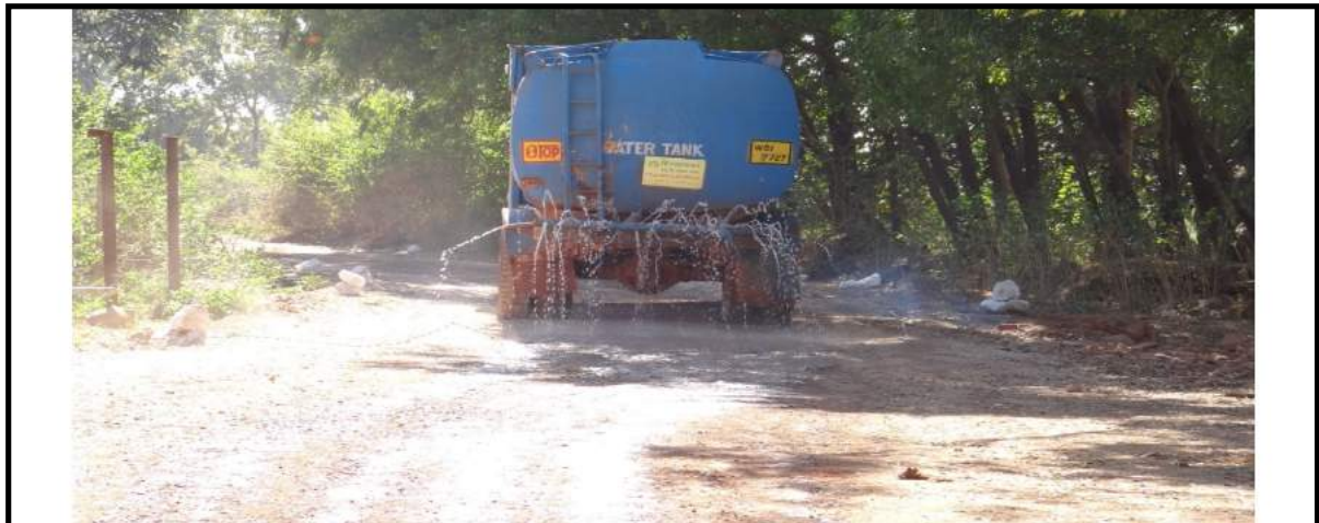
Water Sprinkling at Bagru Mines
