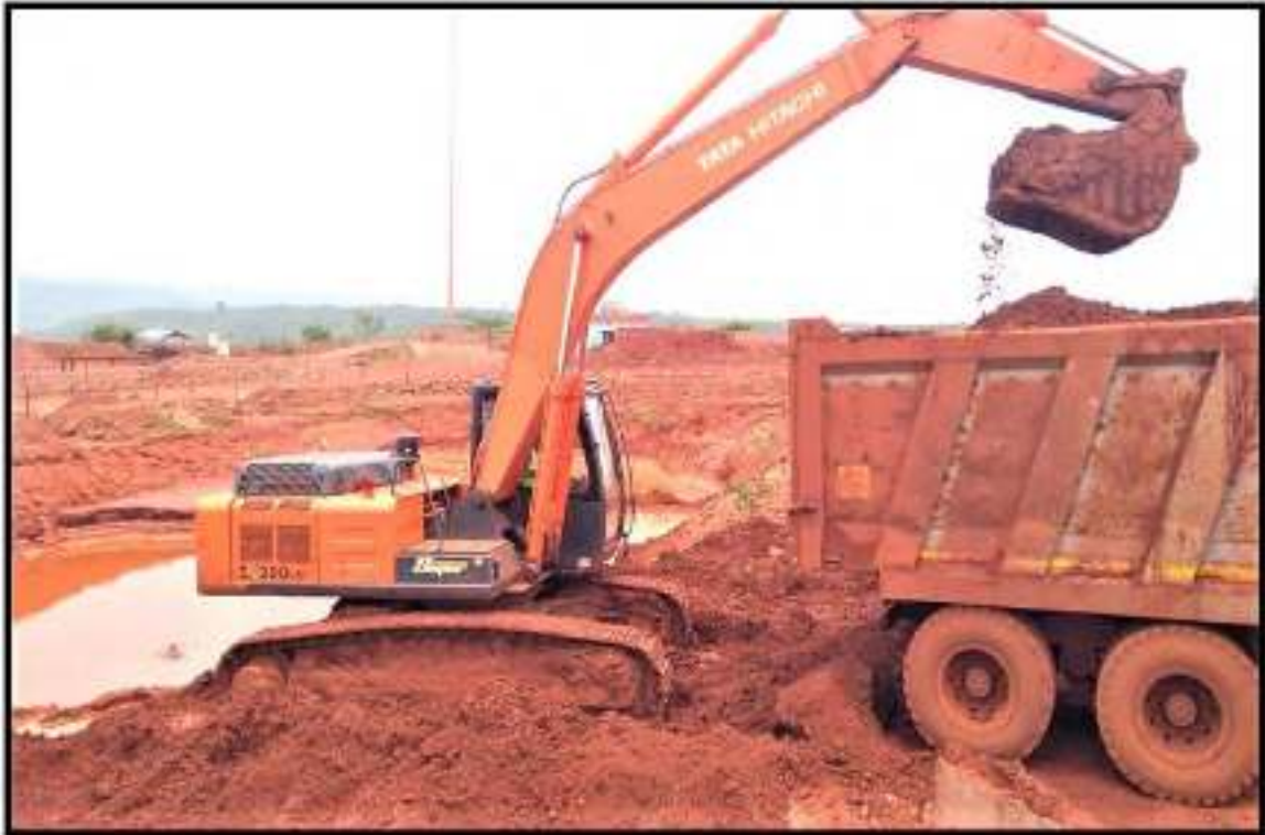
PHOTO 4: Showing Settling Pond Desilting
