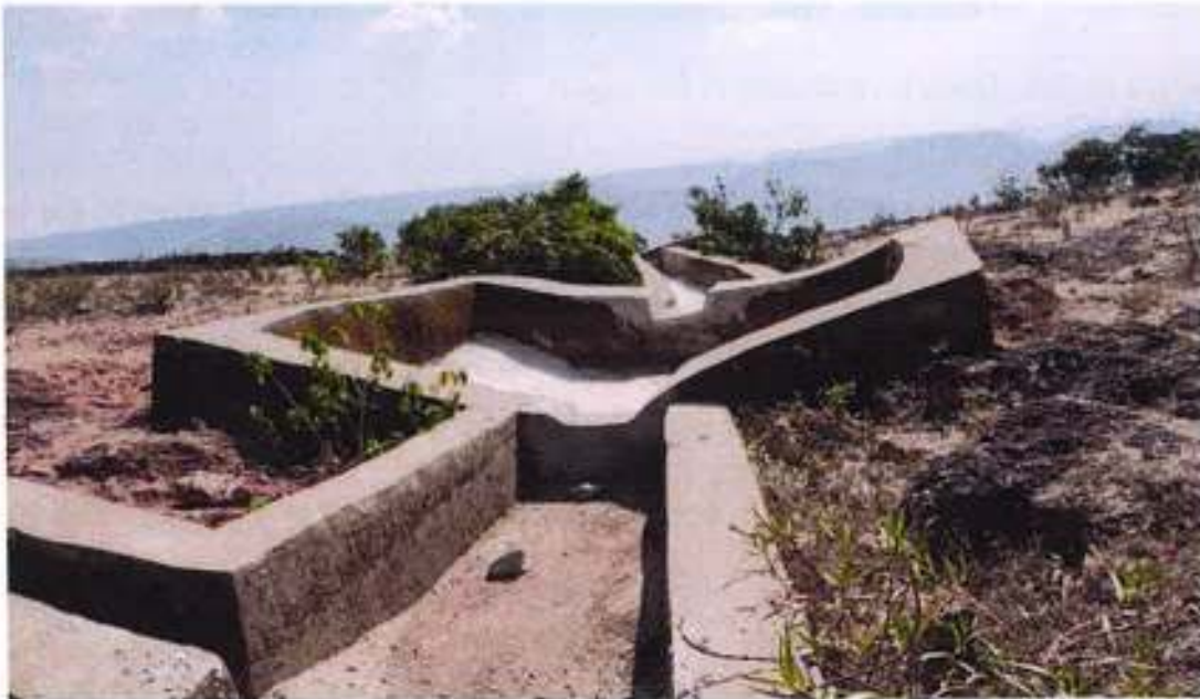
Figure 7: Renovated settling pits
