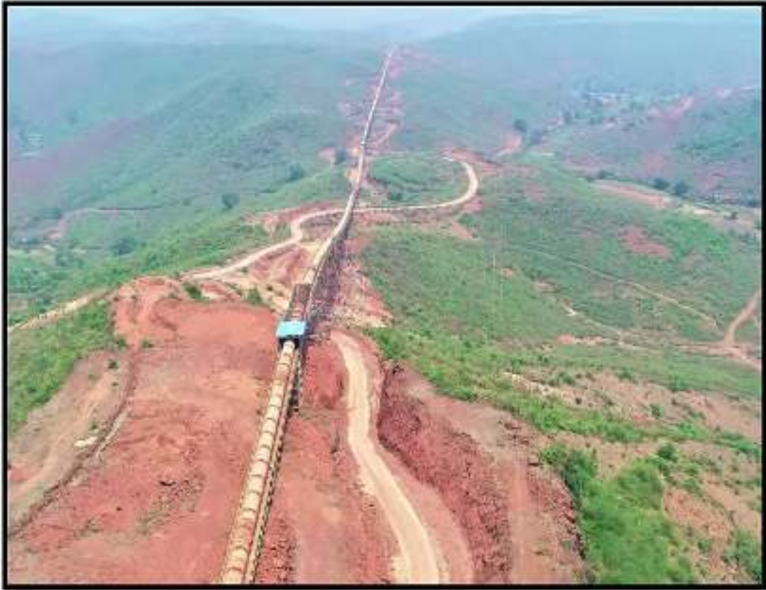
PHOTO 12: Showing Covered Long distance Conveyor
