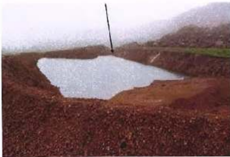
Figure 8: Settling pond near Rayagada dump.
