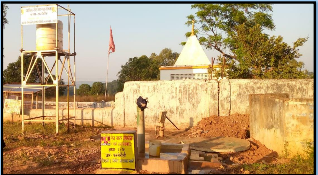
A View of Pond and RWHT Structure
