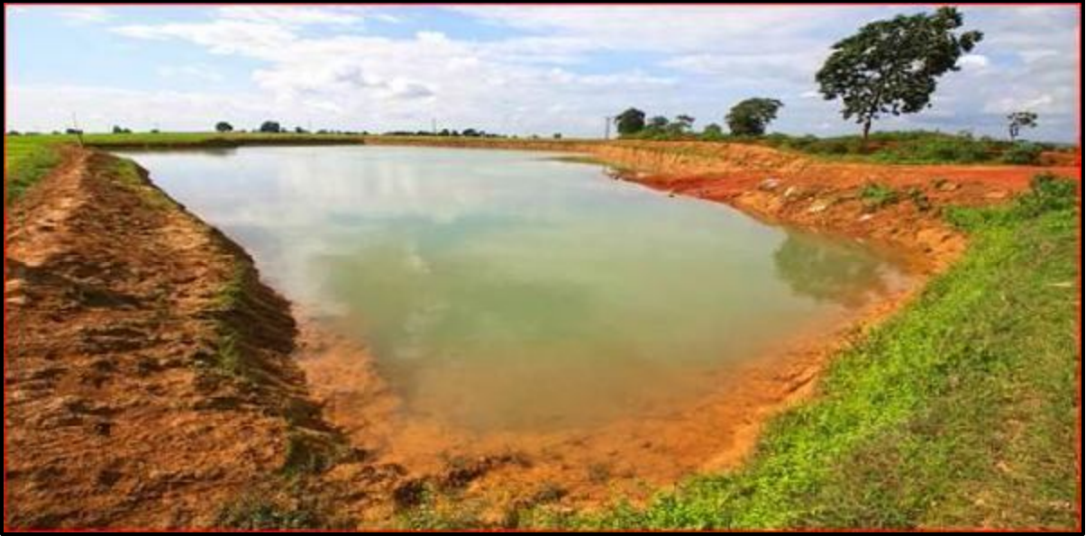
(Rainwater harvesting pond)
