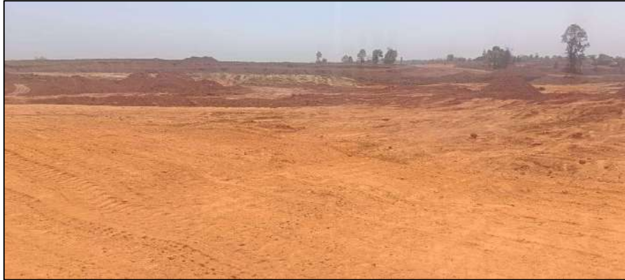
Top Soil Spreading for Backfilling
