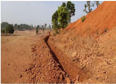
Photographs of garland drains and parapet walls
