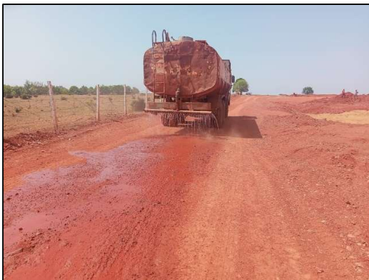
Water Sprinkling in haul road
