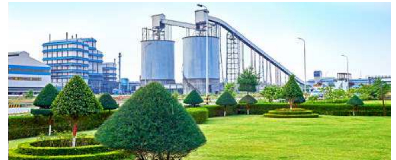
A view of the Mahan Smelter, The plant was conferred Mission Energy's 'Best Energy Efficient' Plant in coal preparation category (2021)
