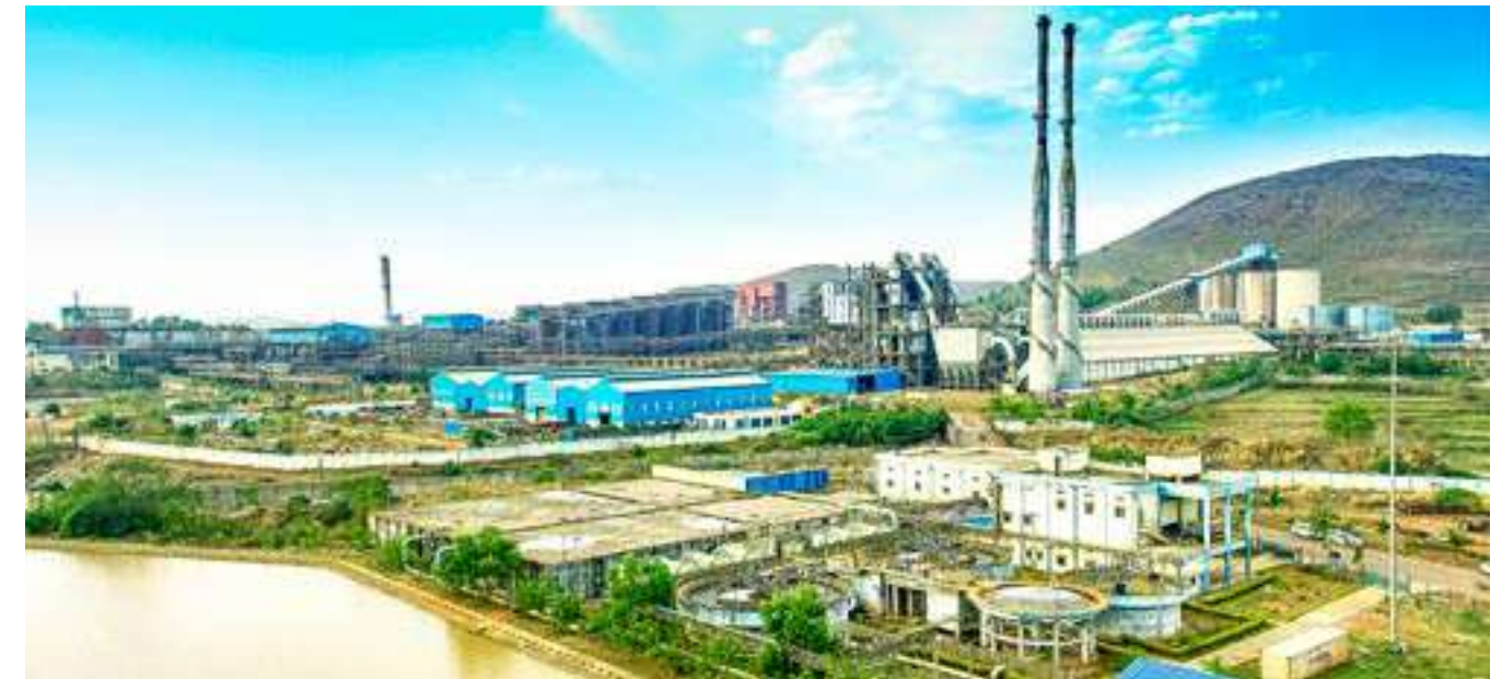
A view of our flat-rolled products plant at Hirakud. Hindalco has implemented the Energy and Carbon Technical Standard and ISO 50001 to reduce energy consumption
