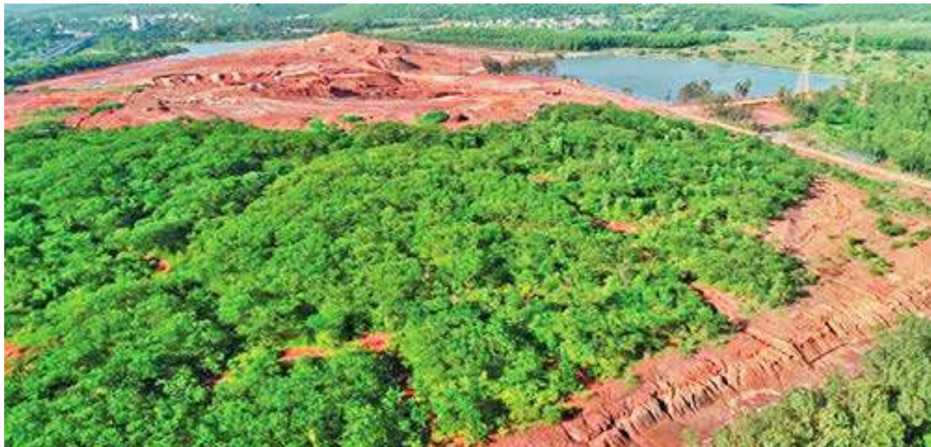
In partnership with TERI, the Belagavi Team successfully re-vegetated the red mud dam at the location to reduce fugitive emissions and make it strong enough to support ecosystems
