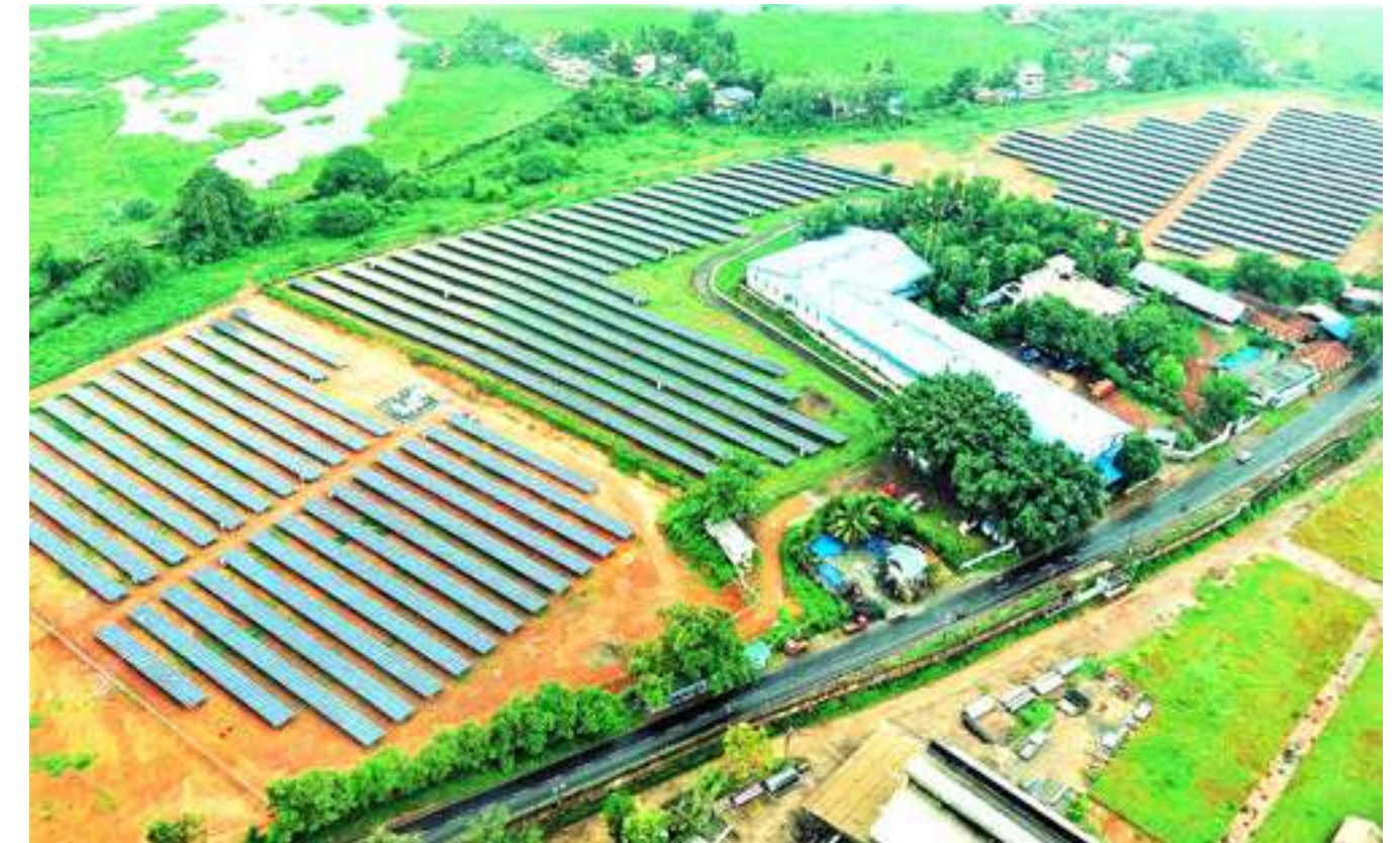
Solar Plant at Alupuram
