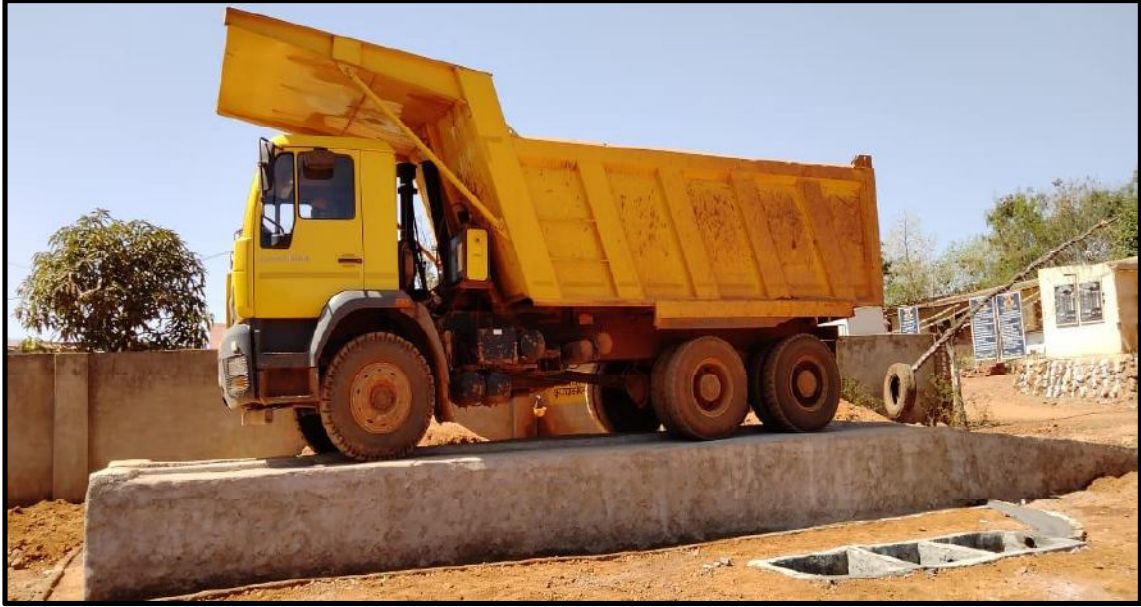
(Pic: Washing platform and oil & grease trap)
