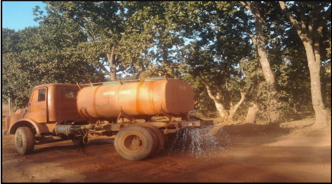
(Pic: Water sprinkling on mines haul road)
