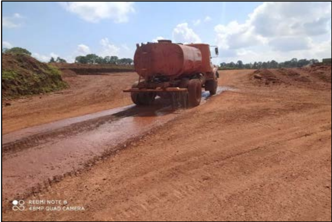
Pic: Water sprinkling on mines haul road.
