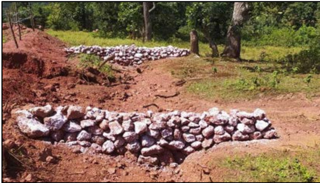
Retaining wall to prevent solid wash-off
