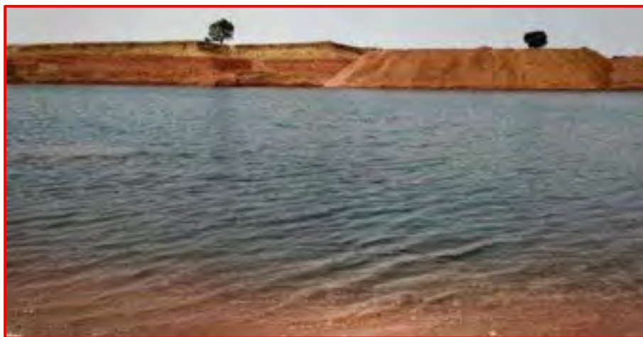
Rainwater Harvesting Pond
