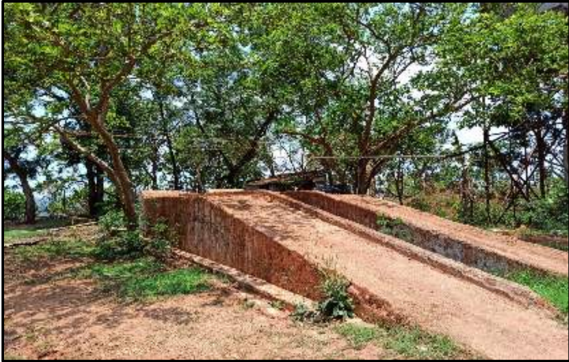
(Photograph of Oil and Grease Trap)
