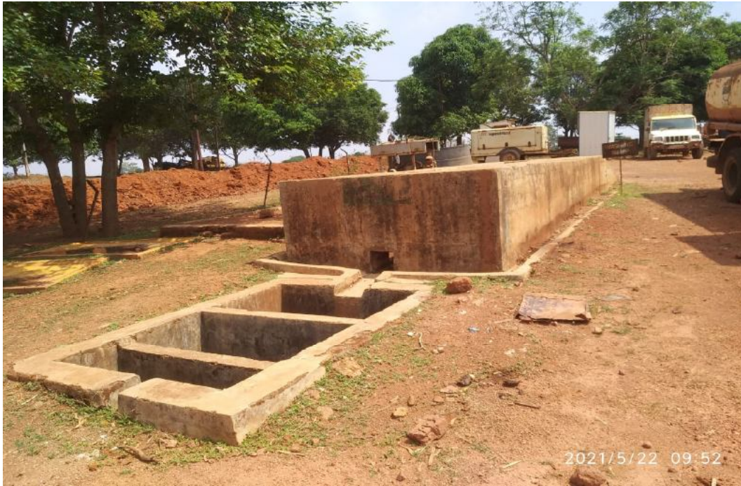
(Washing Ramp and Oil and grease trap)
