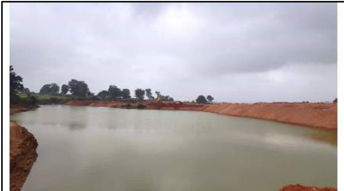
(Rainwater harvesting pond)
