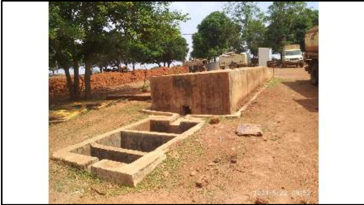
(Washing platform and oil & grease trap)
