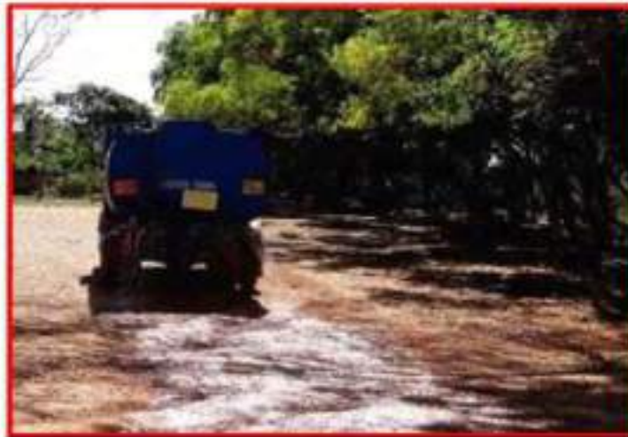
Water sprinkling through tanker
