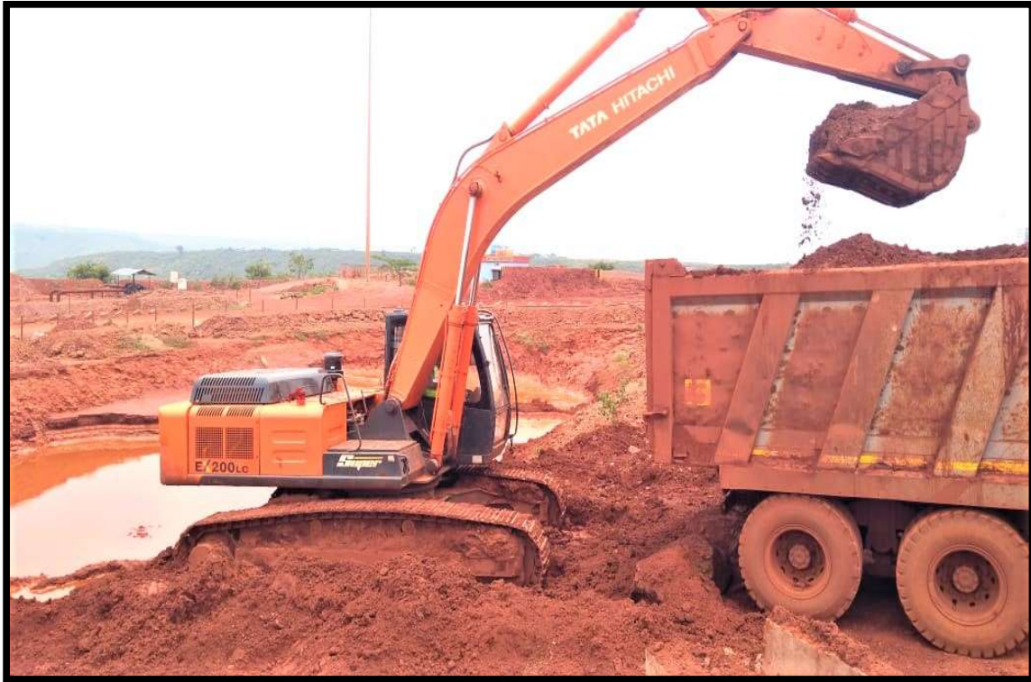
PHOTO 4: Showing Settling Pond Desilting
