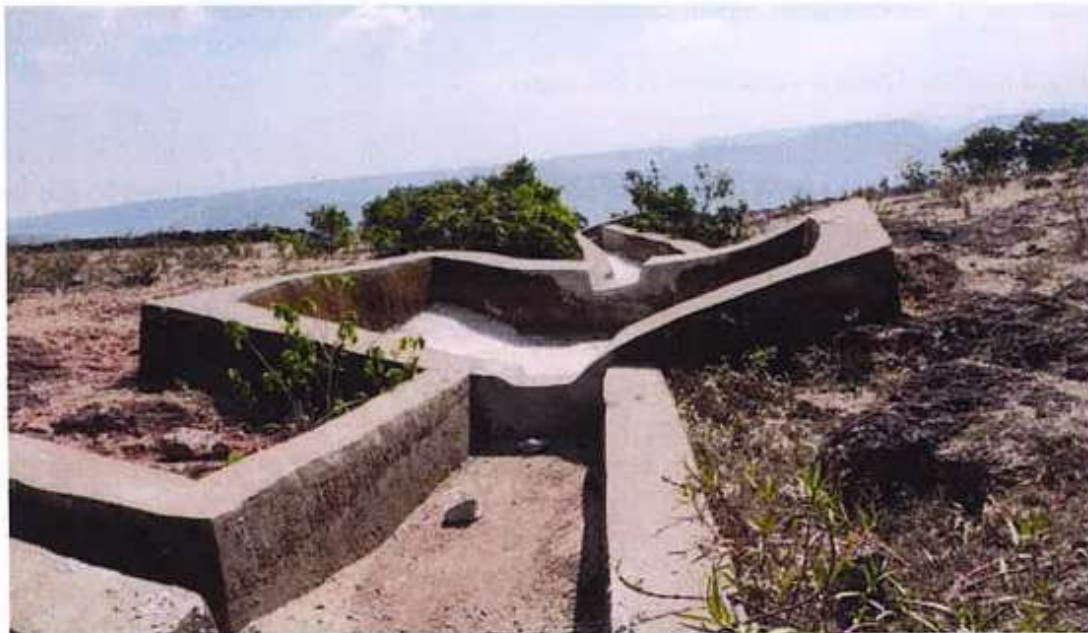
Figure 7: Renovated settling pits
