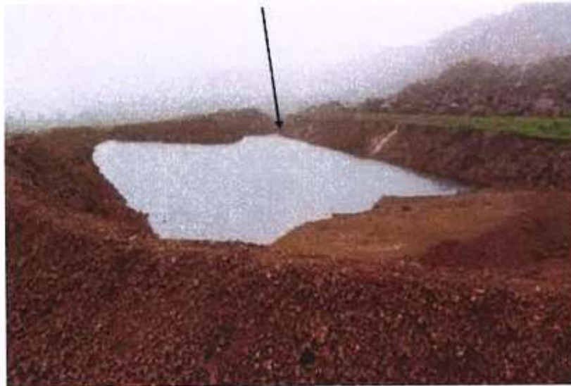
Figure 8: Settling pond near Rayagada dump.
