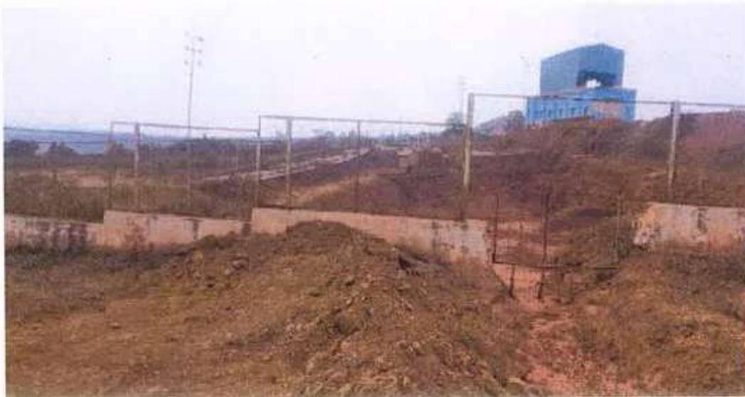
Figure 10: Fencing around the settling pit
